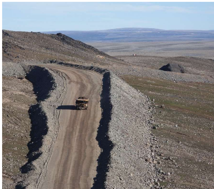
Aerial View of the Haul Road (August 2022)
