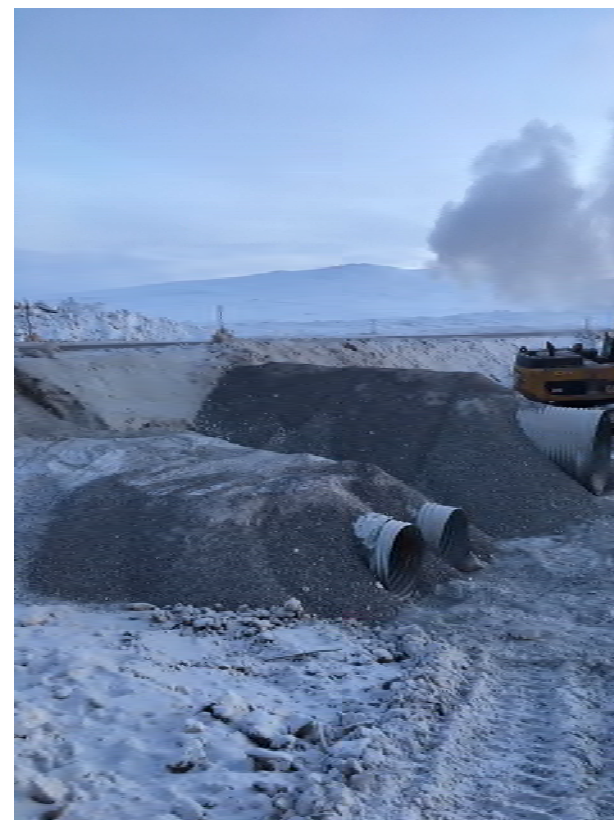
Figure 8. BG04 construction activities
