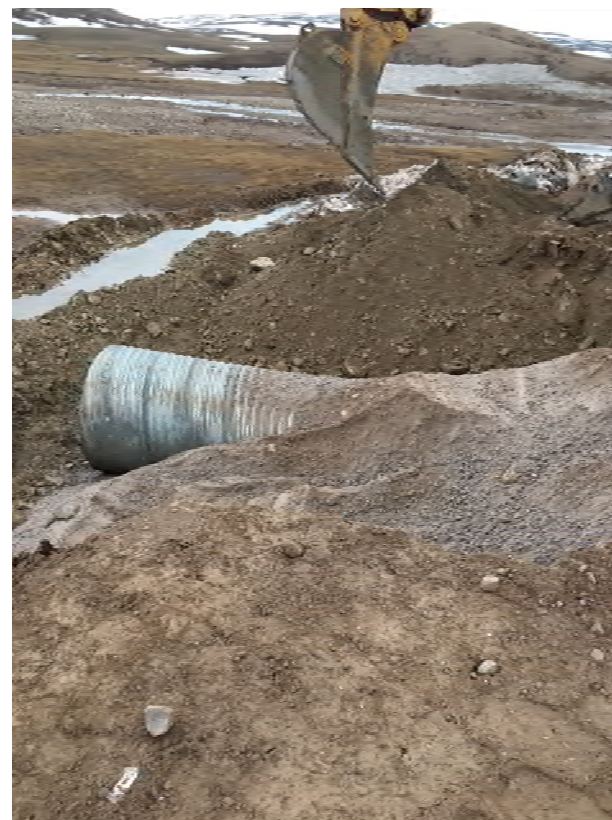
Figure 2. CV079 construction activities
