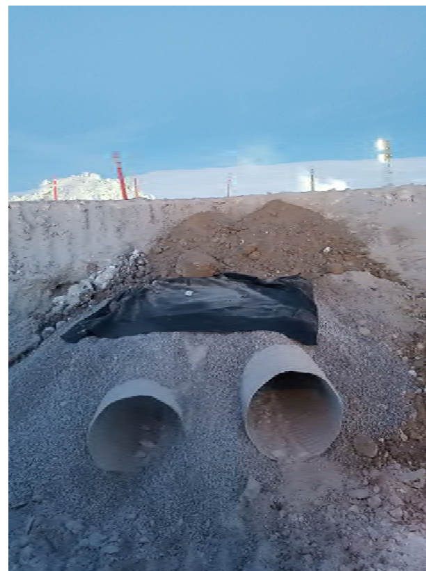
Figure 8. CV224 construction activities
