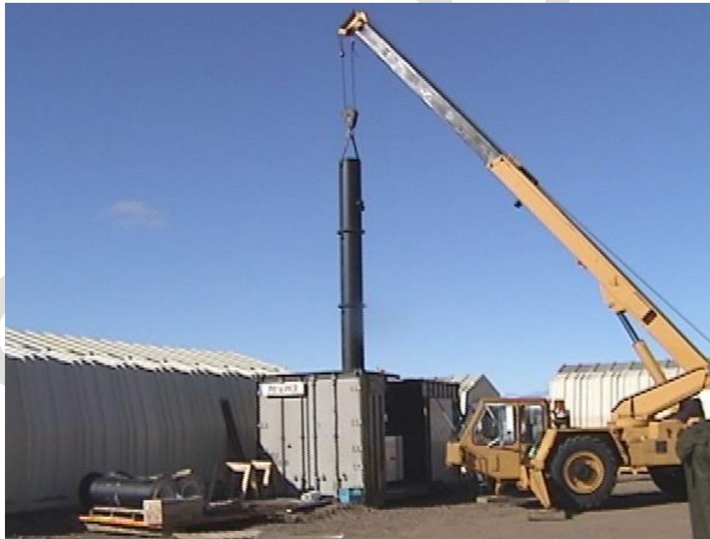
This is a Sample Photo only of Erection of the Stack Sections
