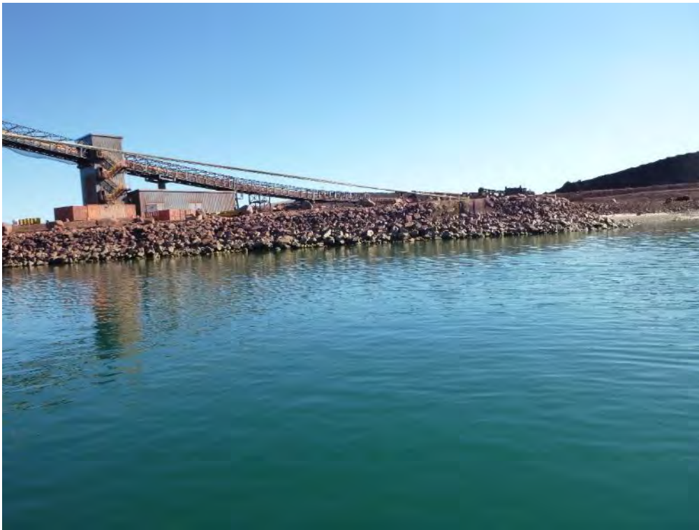
Photo 1 – Station SW-1, west of Ore Dock.
