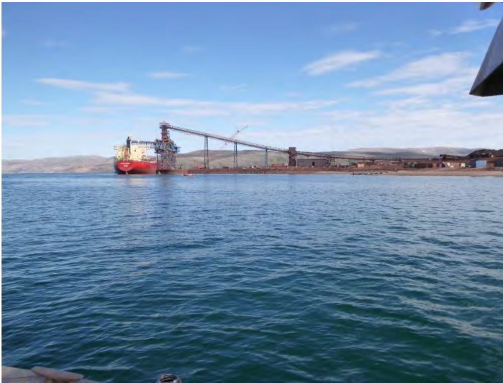
Photo 9 – Station SW-4, looking east towards Ore Dock.
