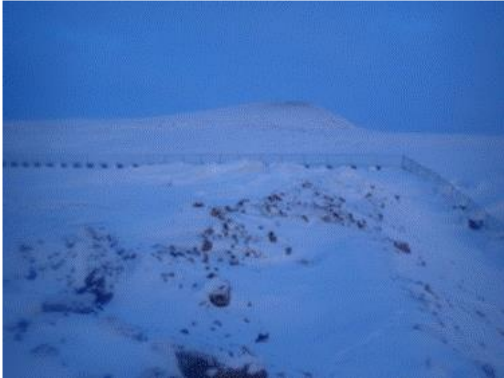
Photo 12-1. View of recently installed fencing enclosing the landfill site to minimize windblown debris escapement and wildlife interactions at the Mary River Project.
