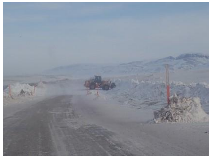
Photo 10-7. View of snowbank management in progress along Tote Road to facilitate wildlife crossing and improve drivers' visibility (near km 72; April 11, 2020).
