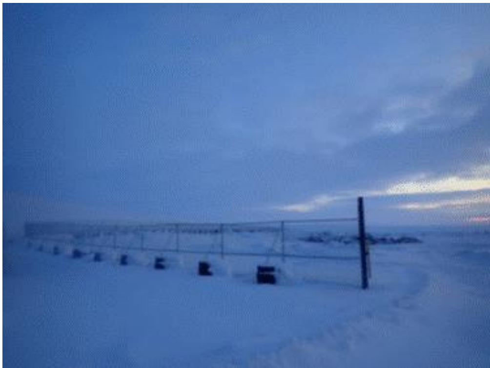
Photo 12-2. View of the entrance to the landfill site with recently installed fencing at the Mary River Project.
