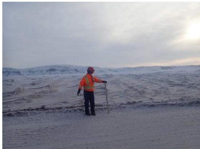
Photo 10-8. View of a snowbank that has been pushed back and feathered along Tote Road to facilitate wildlife crossing and improve drivers' visibility (km 76.7; April 11, 2020).
