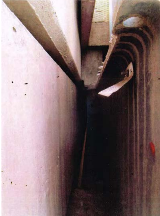
Photo 3 - South Abutment – SE Corner
