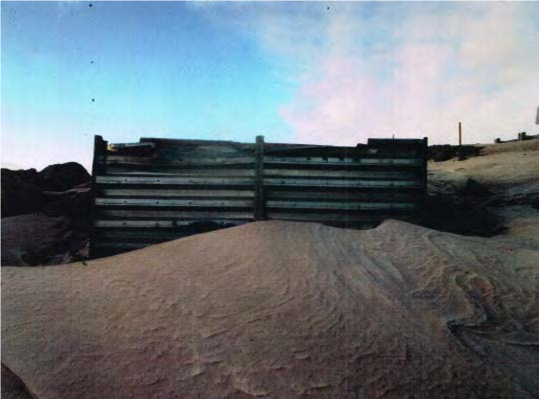
Photo 5 – North Abutment (Former Shipping Container Bridge)
