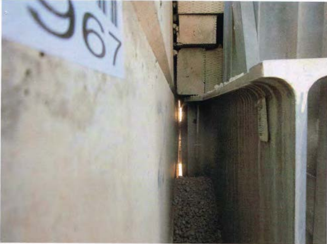
Photo 1 - North Abutment - NW Corner
