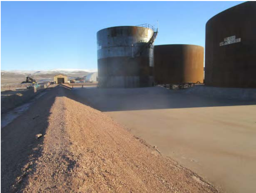
2. Port Site Fuel Tank Farm
