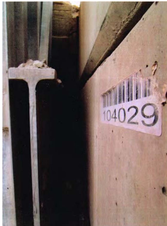
Photo 4 - South Abutment – SW Corner
