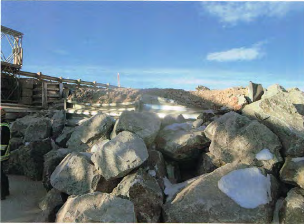
Photo 3 - North Abutment (Former Shipping Container Bridge)
