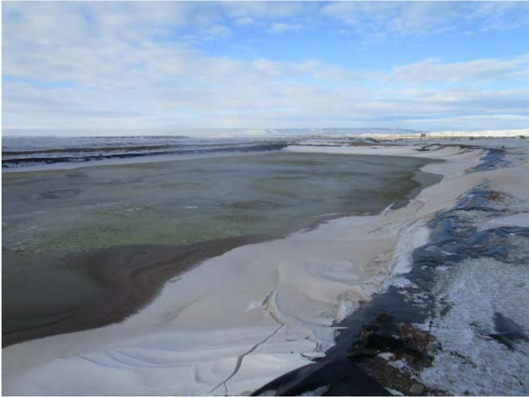
C. PWSP #1 – Repair Liner at Unloading Area
