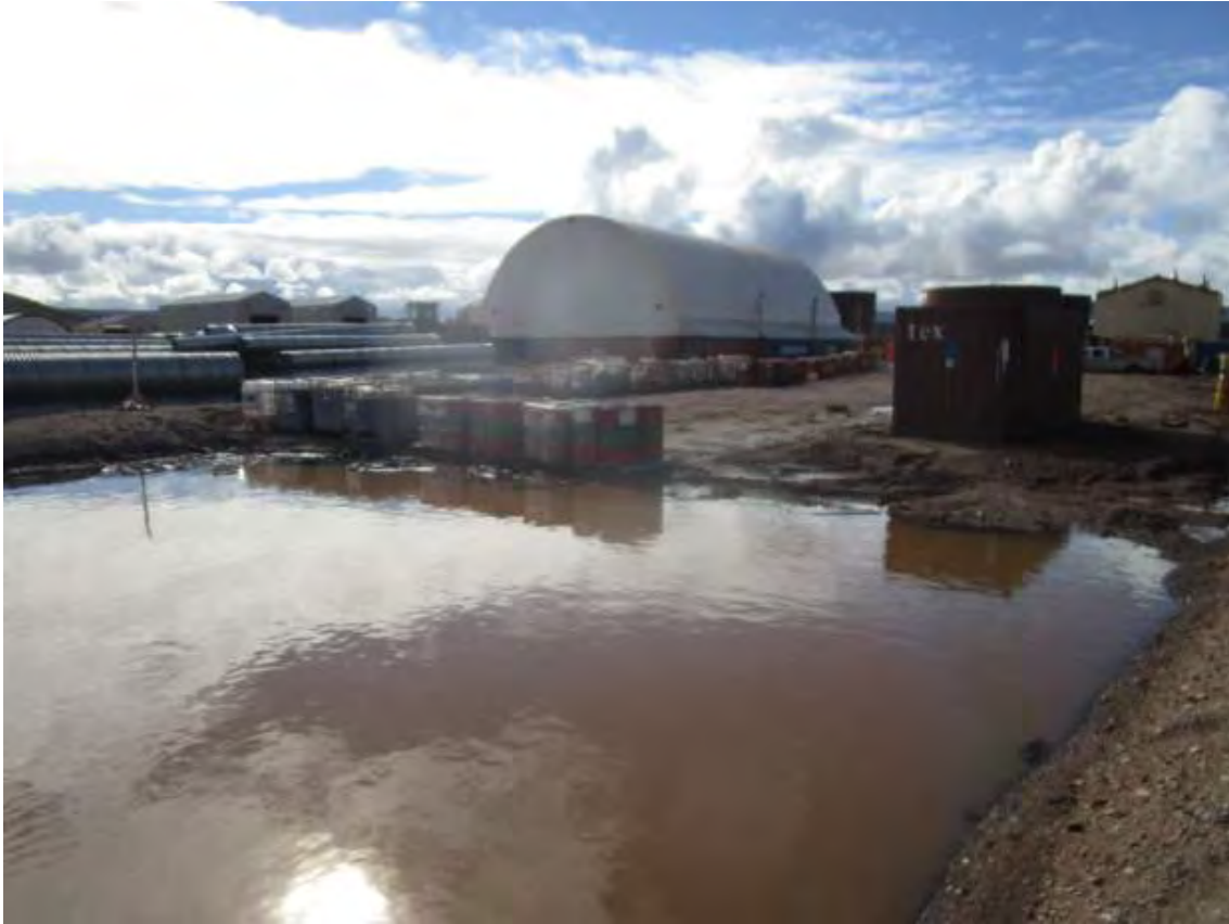
9. Loading Area Contaminated Storage (MP-HWB-1)
