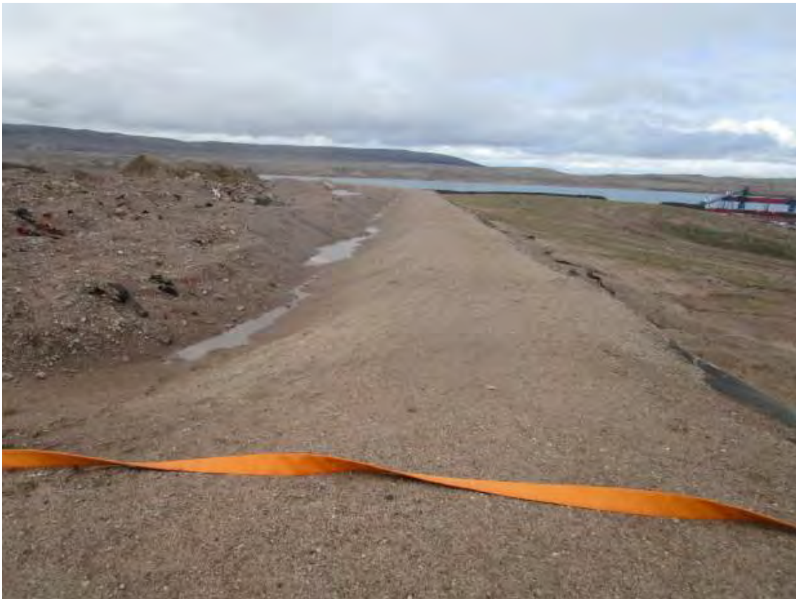
4. Land Farm Containment
