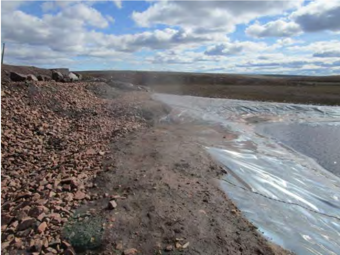
15. Crusher Pad Drainage Containment
