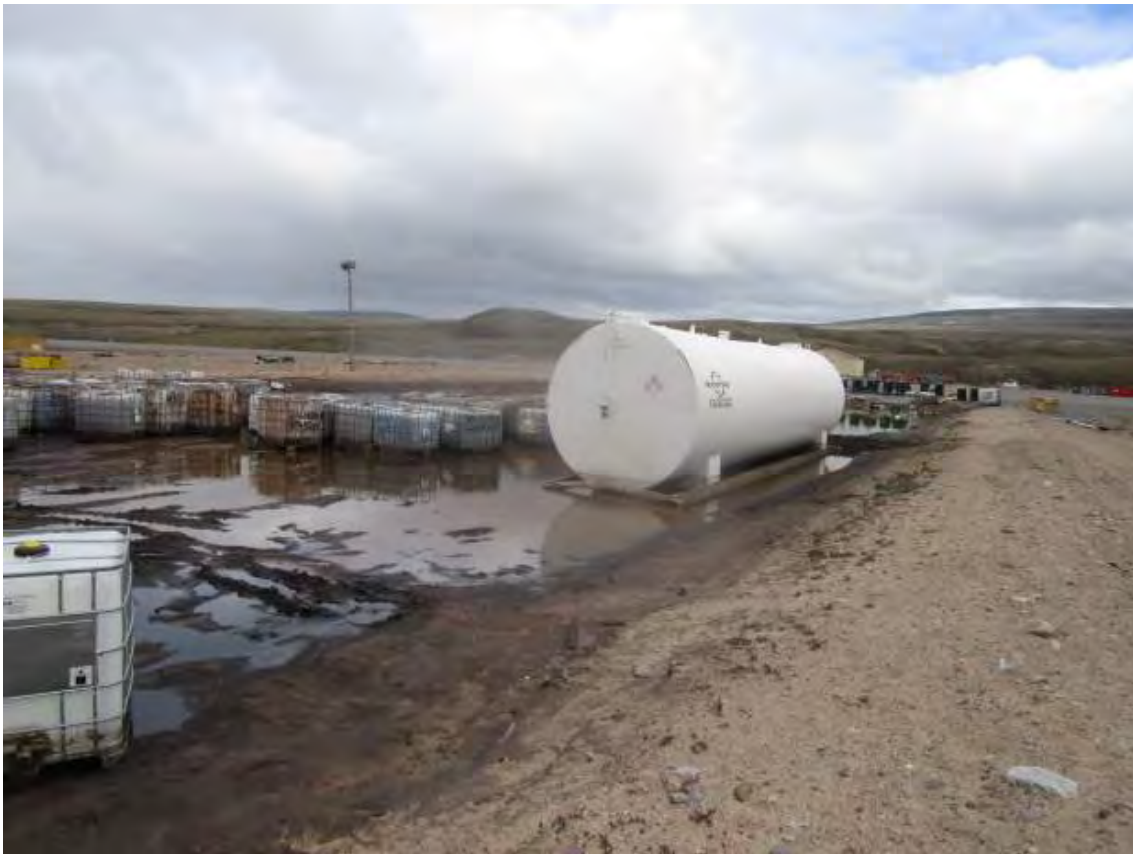
1. Bulk Fuel Storage Facility.
