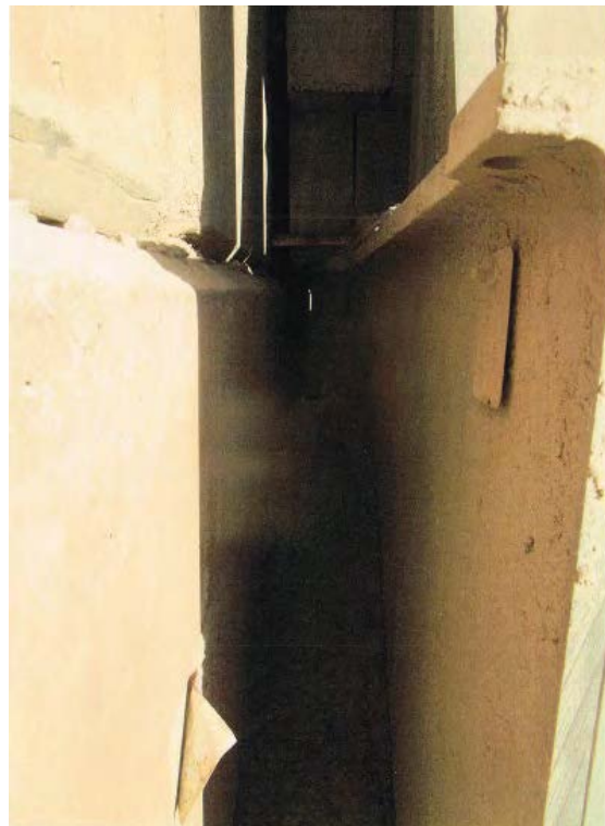
Photo 2 - North Abutment - NW Corner
