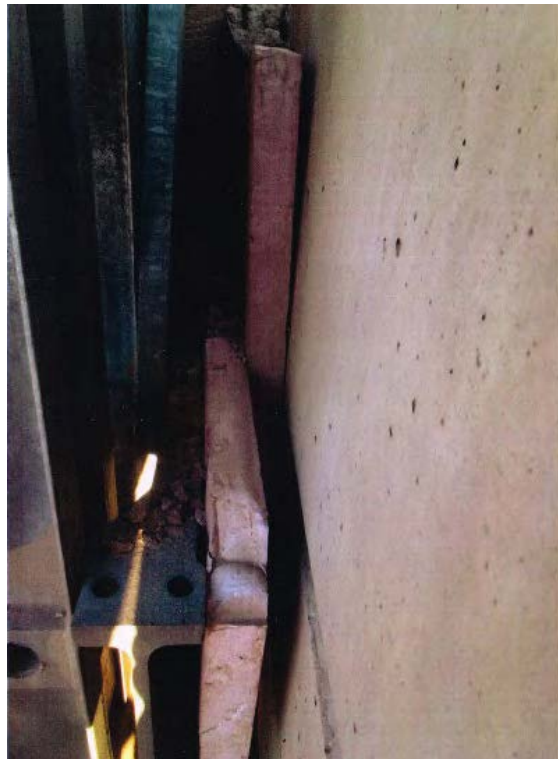
Photo 4 - South Abutment – SW Corner
