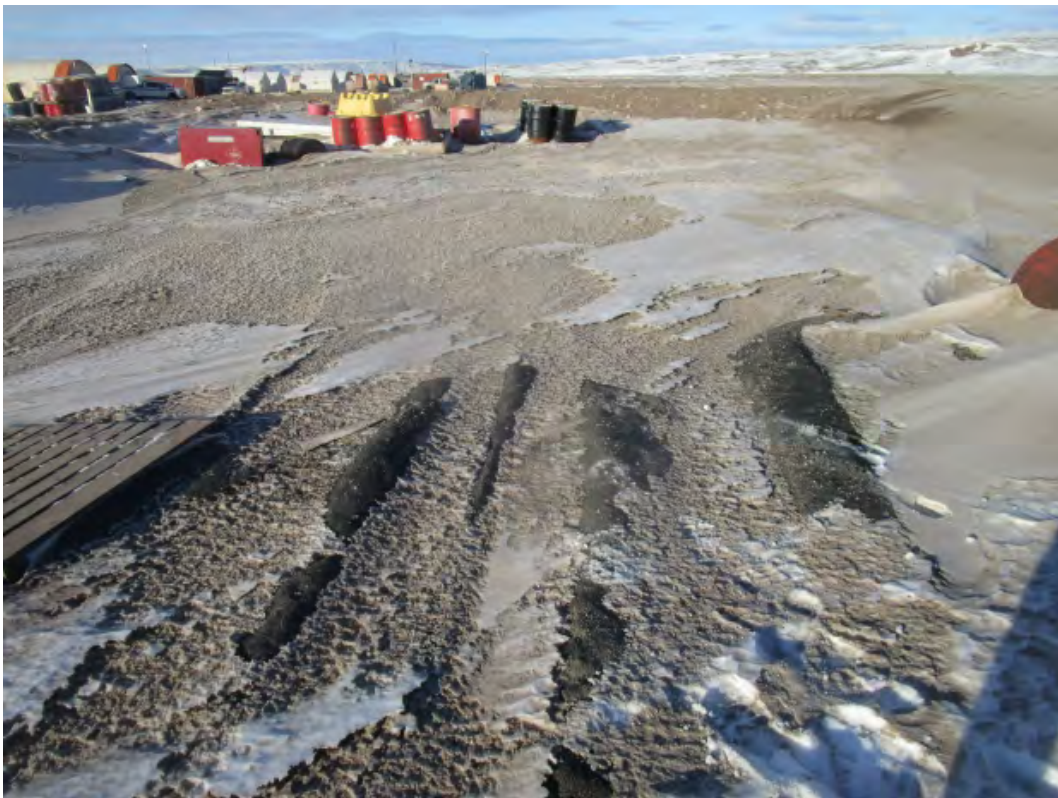
H. MS-HWB-2 – Hazardous Waste Storage – Exposed Liner
