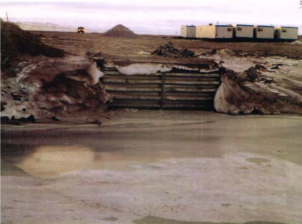
Photo 6 – South Abutment (Former Shipping Container Bridge)
