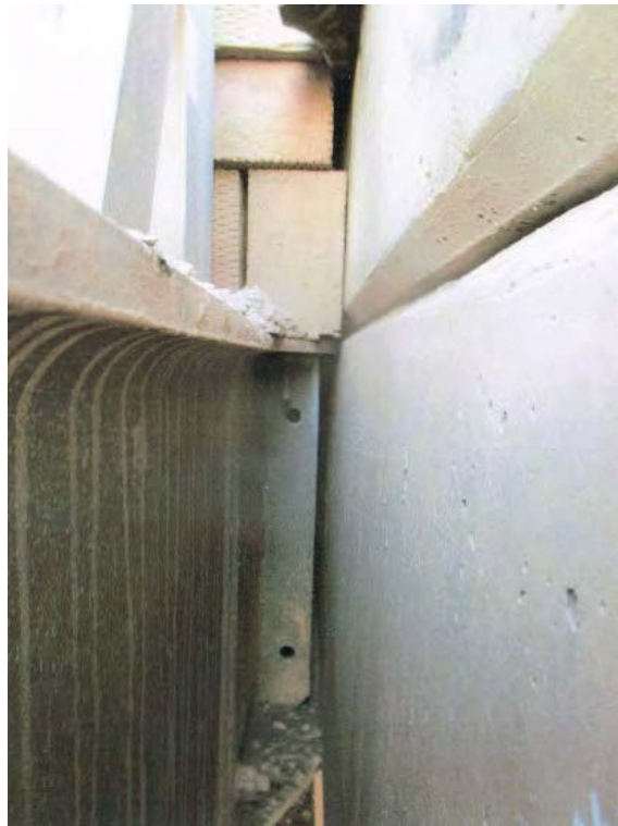
Photo 4 - South Abutment - SW Corner
