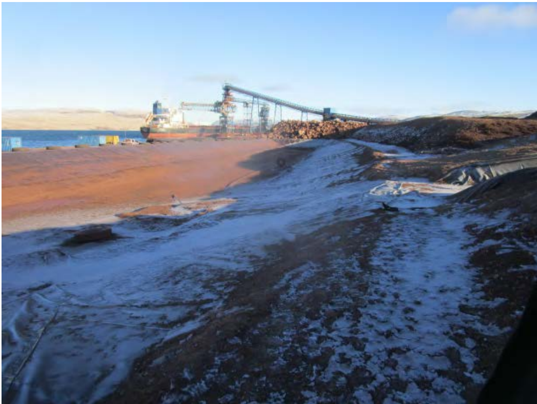
6. Sediment Pond West (MP-06)
