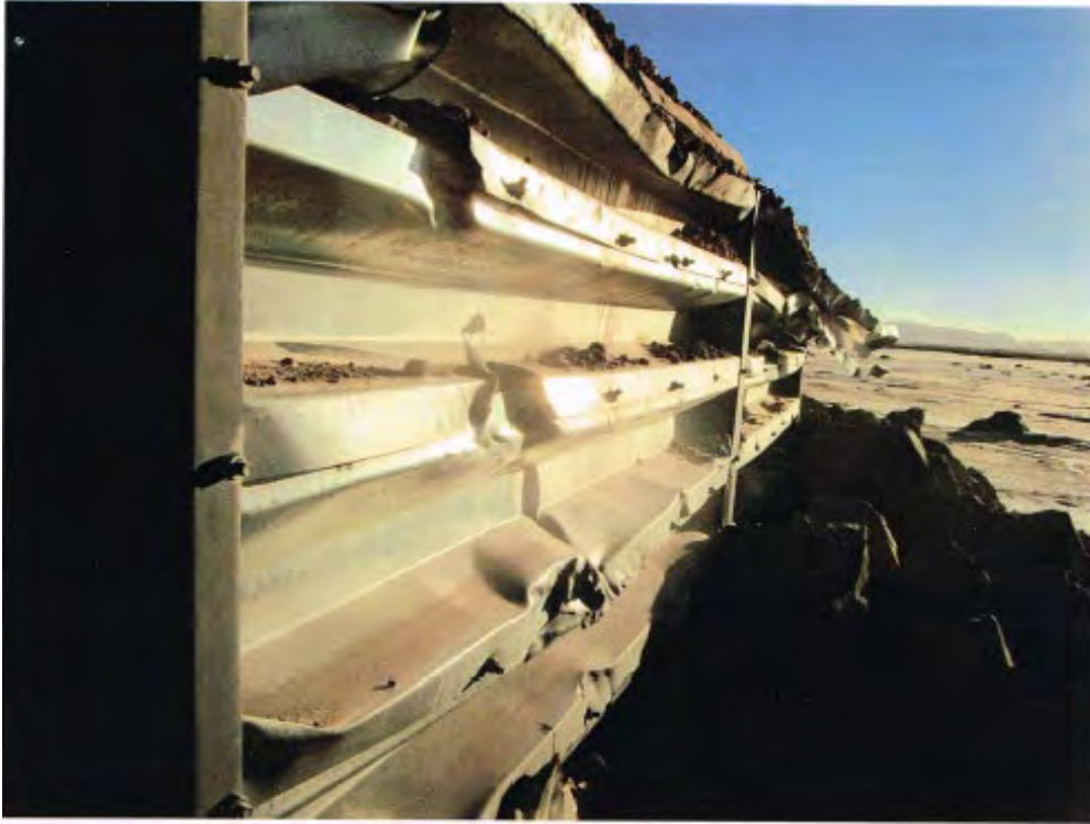
Photo 5 - North Abutment (Former Shipping Container Bridge)
