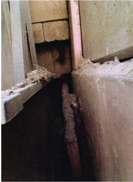
Photo 1 - North Abutment - NE Corner
