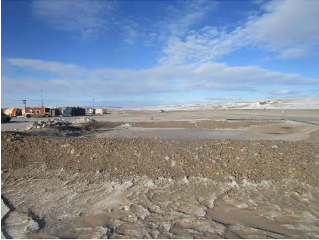
K. Jet Fuel Tank and Pump Containment
