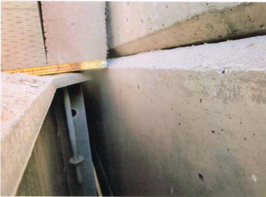
Photo 2 - North Abutment - NE Corner
