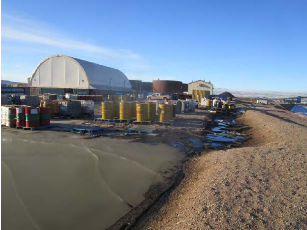
9. Loading Area Contaminated Storage (MP-HWB-1)
