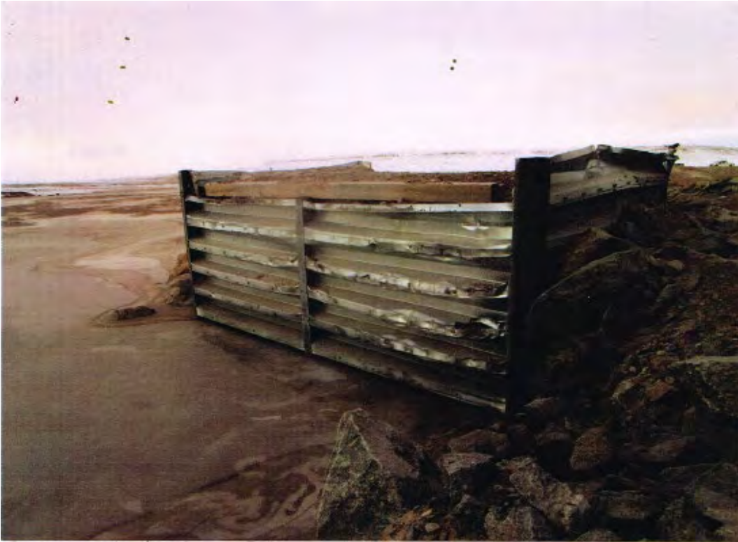
Photo 5 – North Abutment (Former Shipping Container Bridge)
