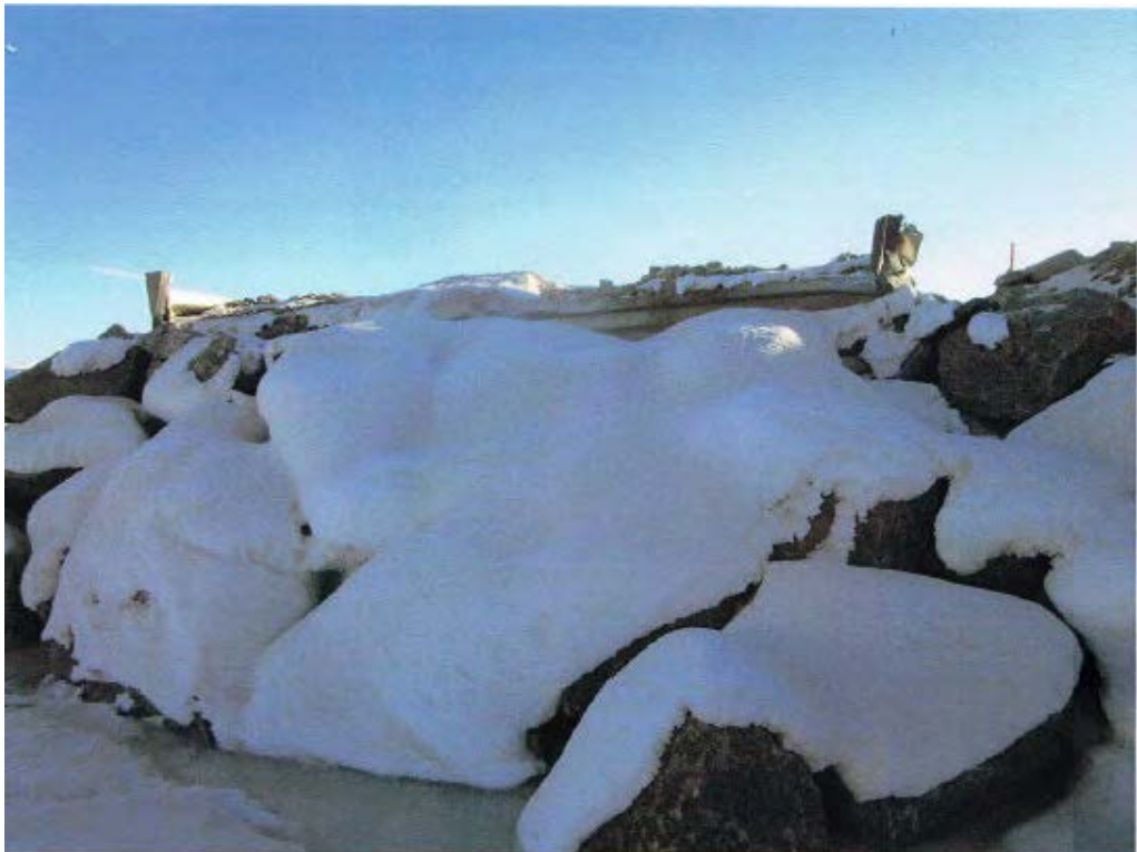
Photo 4 - South Abutment (Former Shipping Container Bridge)
