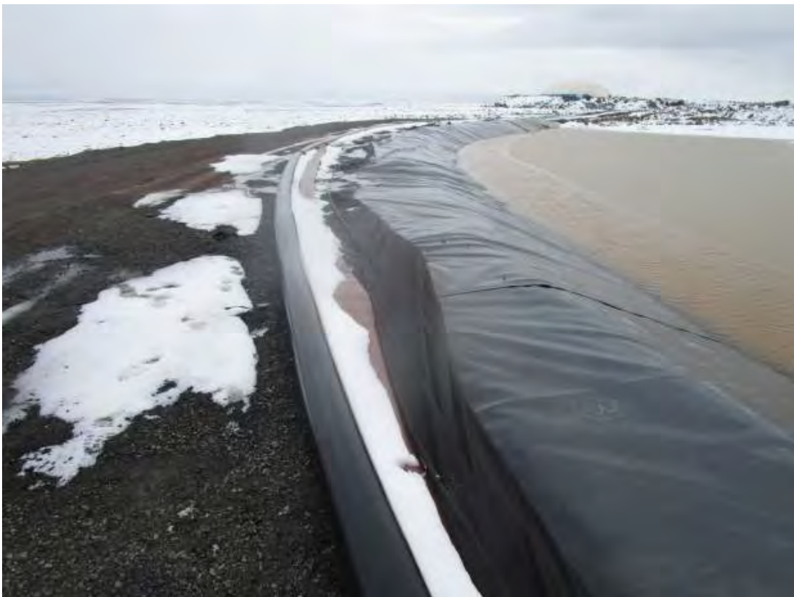
16. Waste Pile Drainage Containment
