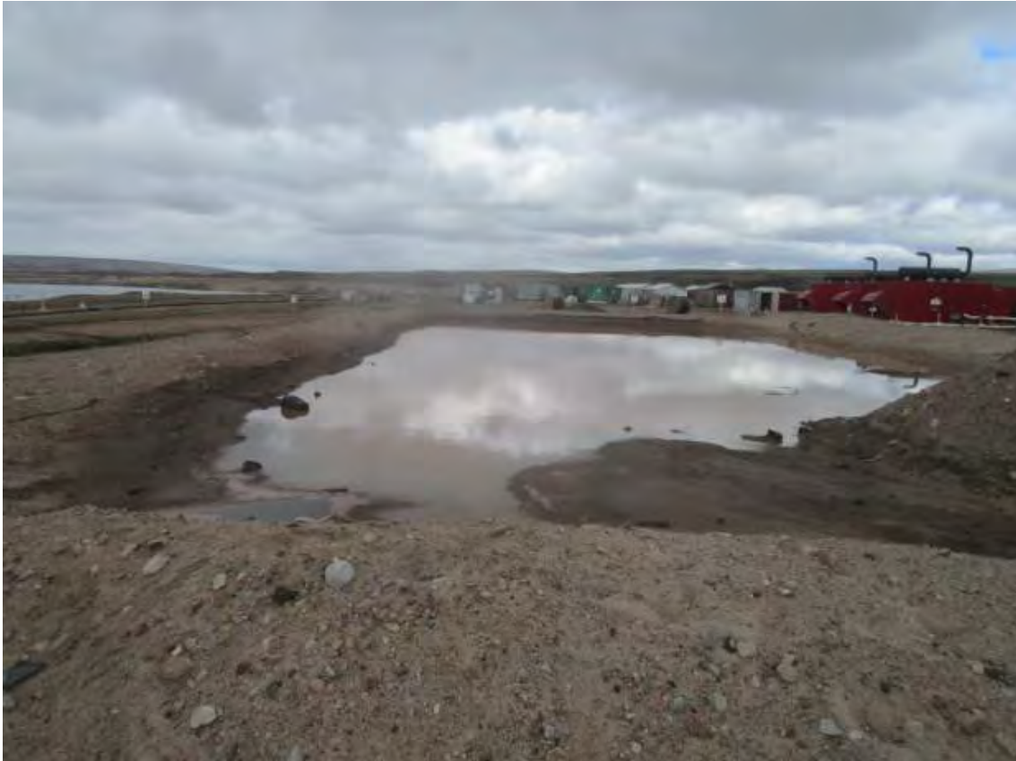
2. Generator Fuel Storage Containment.
