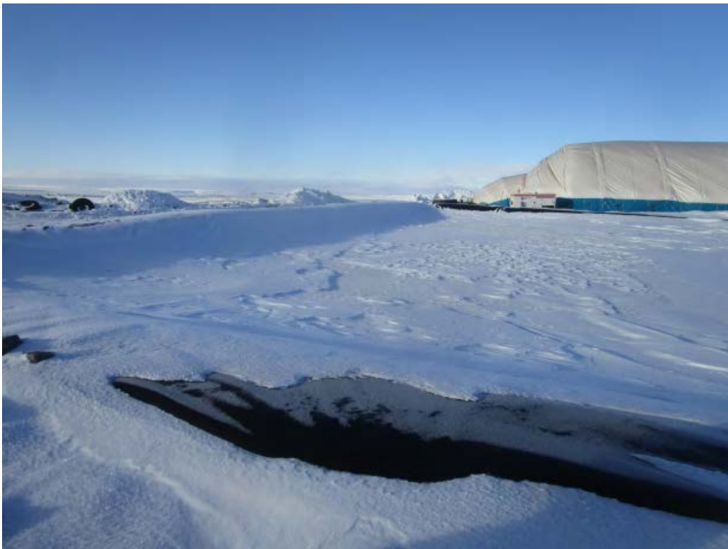
P. Waste Rock Water Treatment System Geotube field
