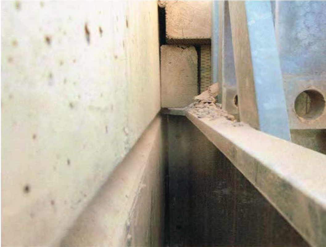
Photo 3 - South Abutment - SE Corner
