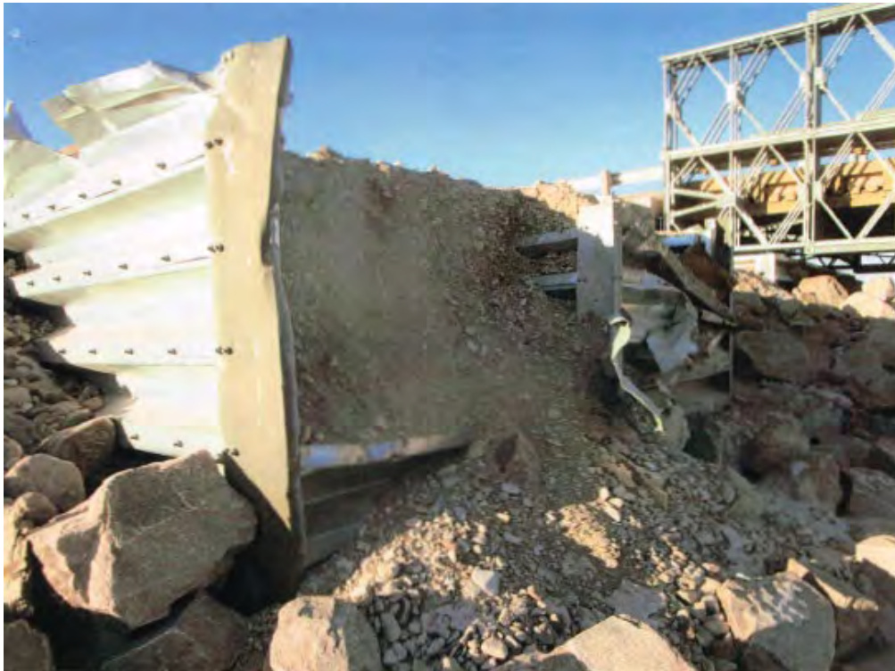
Photo 6 - South Abutment (Former Shipping Container Bridge)
