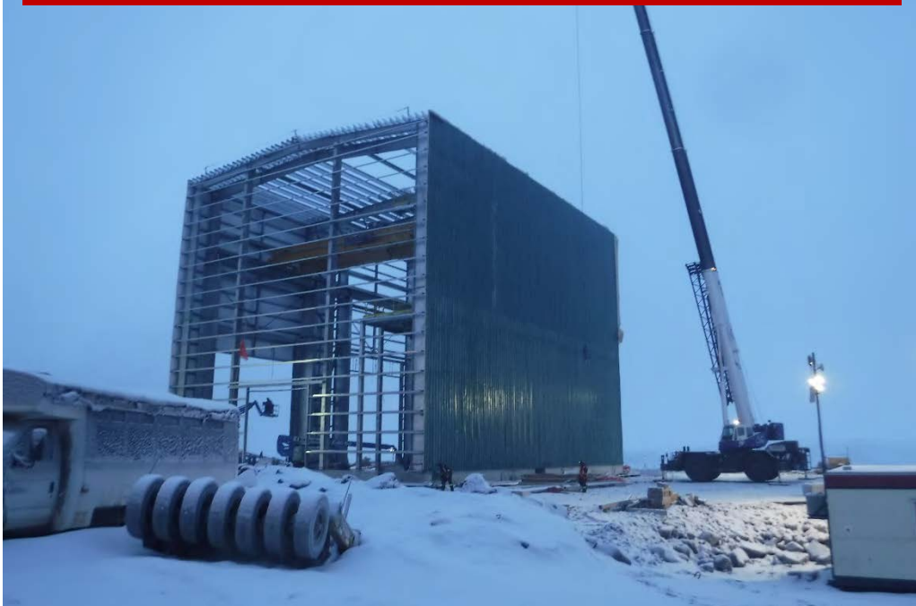
Mine truck shop under construction to accommodate CAT ultra-class trucks
