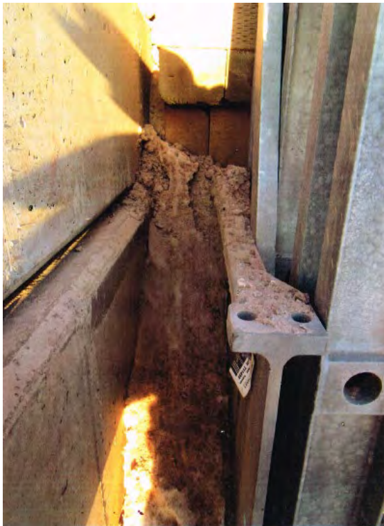
Photo 2 - North Abutment - NW Corner
