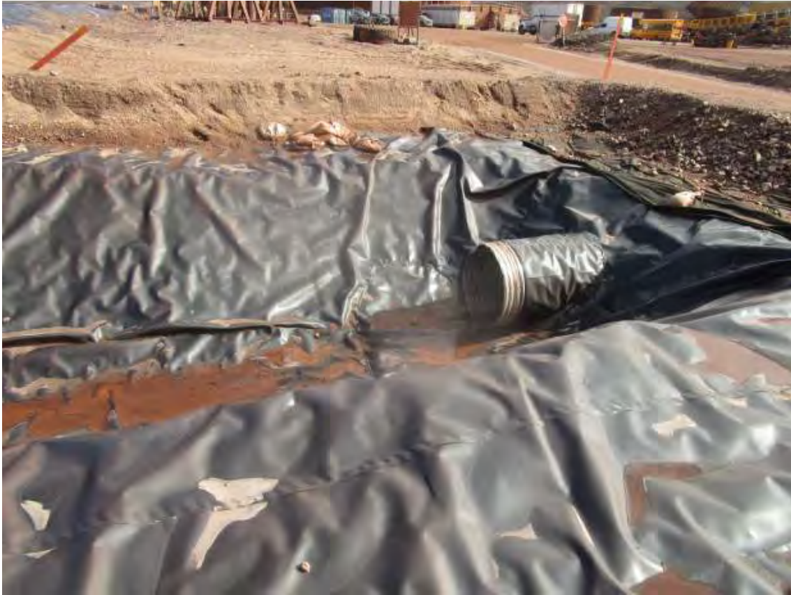
7. Sediment Pond East
