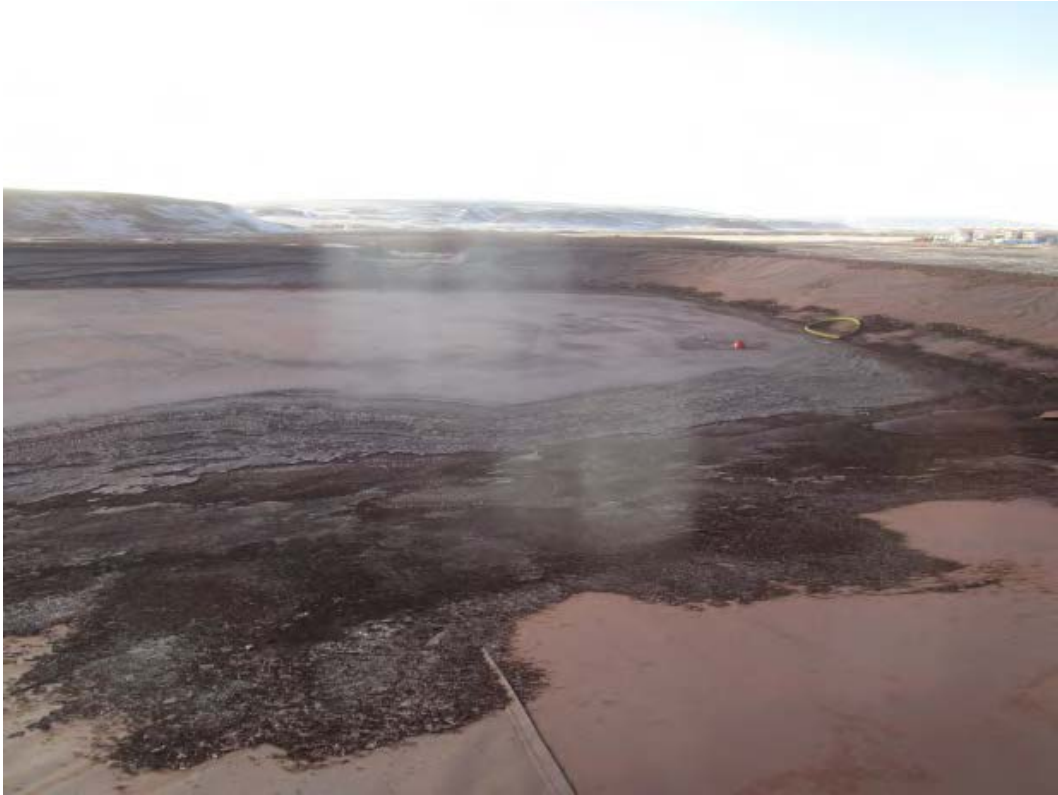
O. Crusher Pad Drainage Containment (MS-06)
