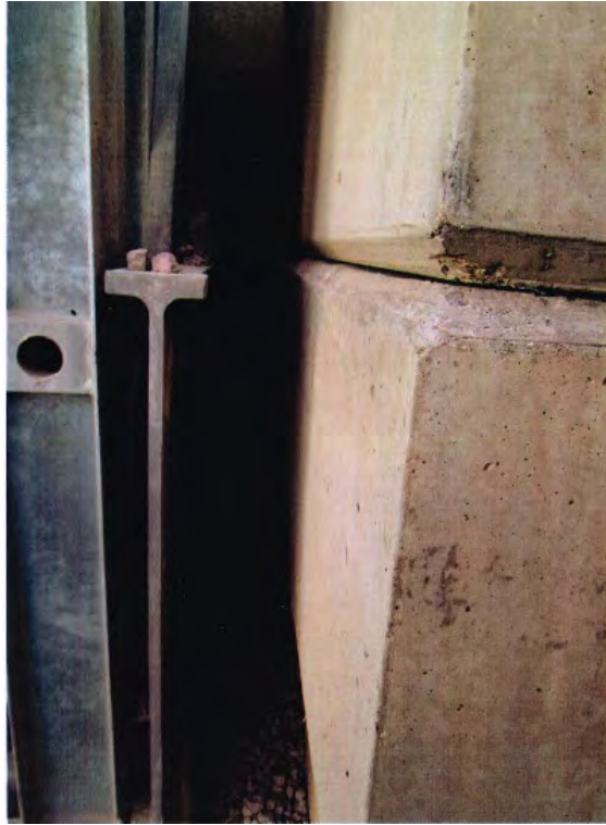
Photo 1 - North Abutment - NE Corner
