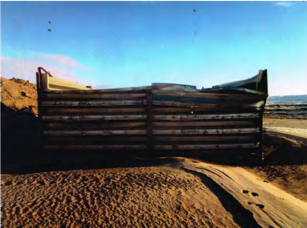
Photo 6 – South Abutment (Former Shipping Container Bridge)
