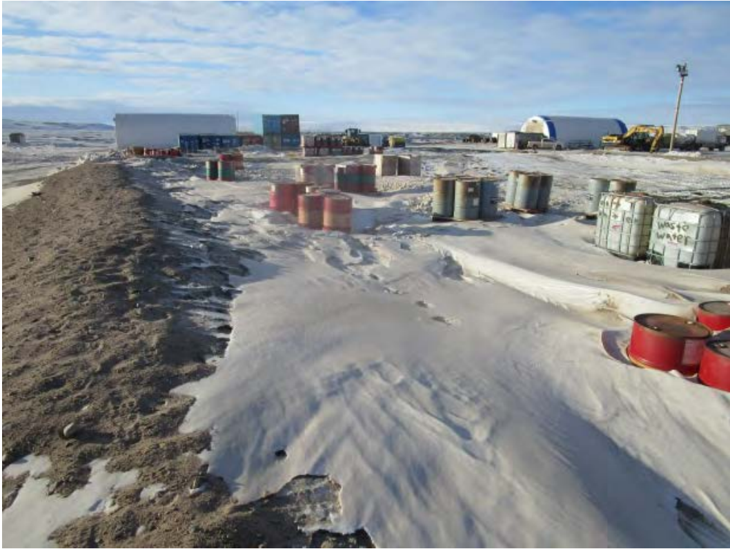
A. Bulk Fuel Storage Facility
