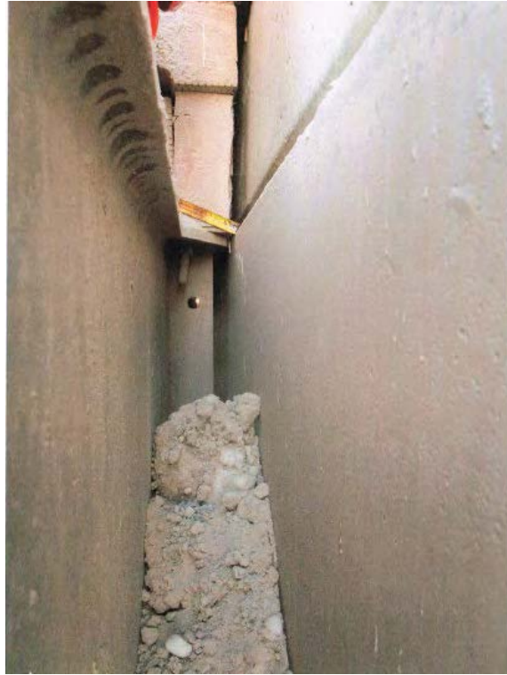
Photo 1 - North Abutment - NE Corner
