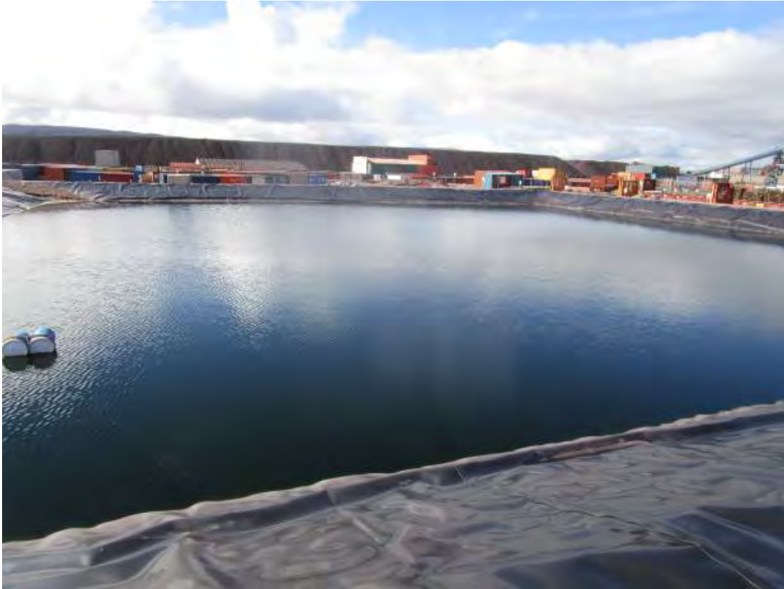
3. Polishing/Waste Stabilization Pond (PWSP)
