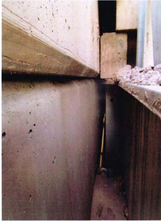
Photo 3 - South Abutment – SE Corner
