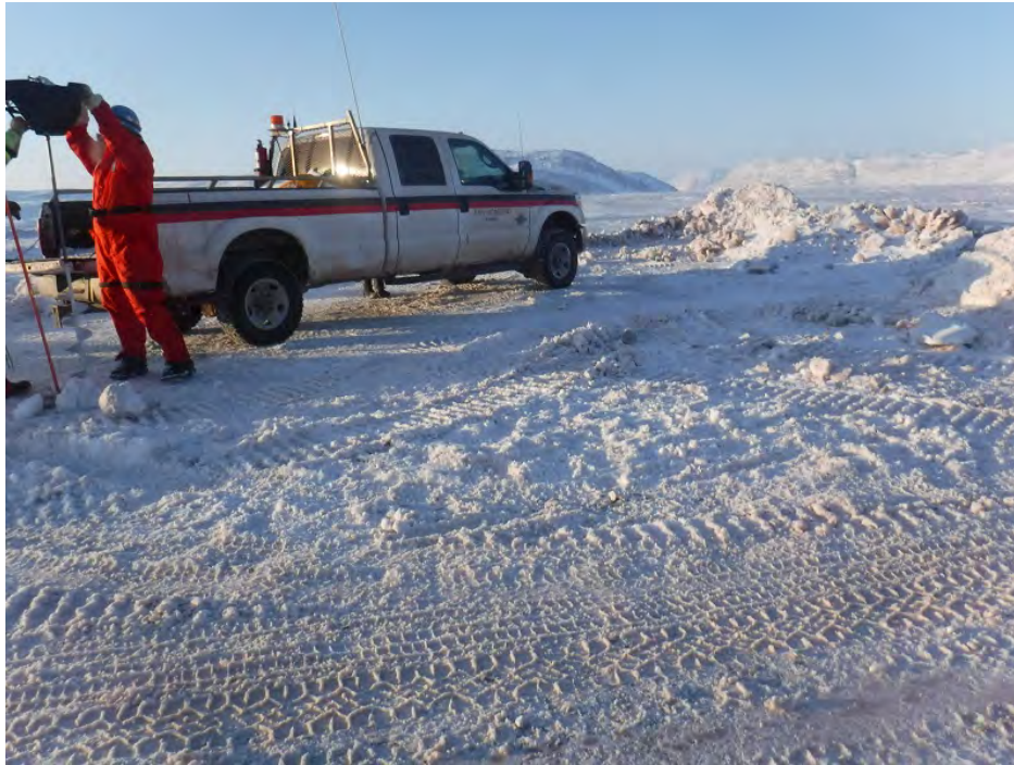
PHOTO 3 - Post-Drilling Conditions at CPT-03, April 2018
