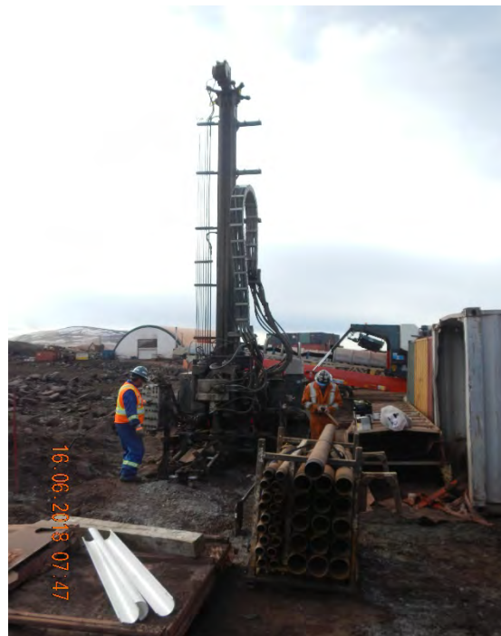
PHOTO 2 - Drilling Conditions at BH18-TW-01, June 2018
