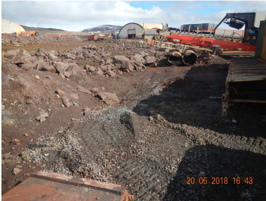
PHOTO 3 - Post-Drilling Conditions at BH18-TW-01, June 2018
