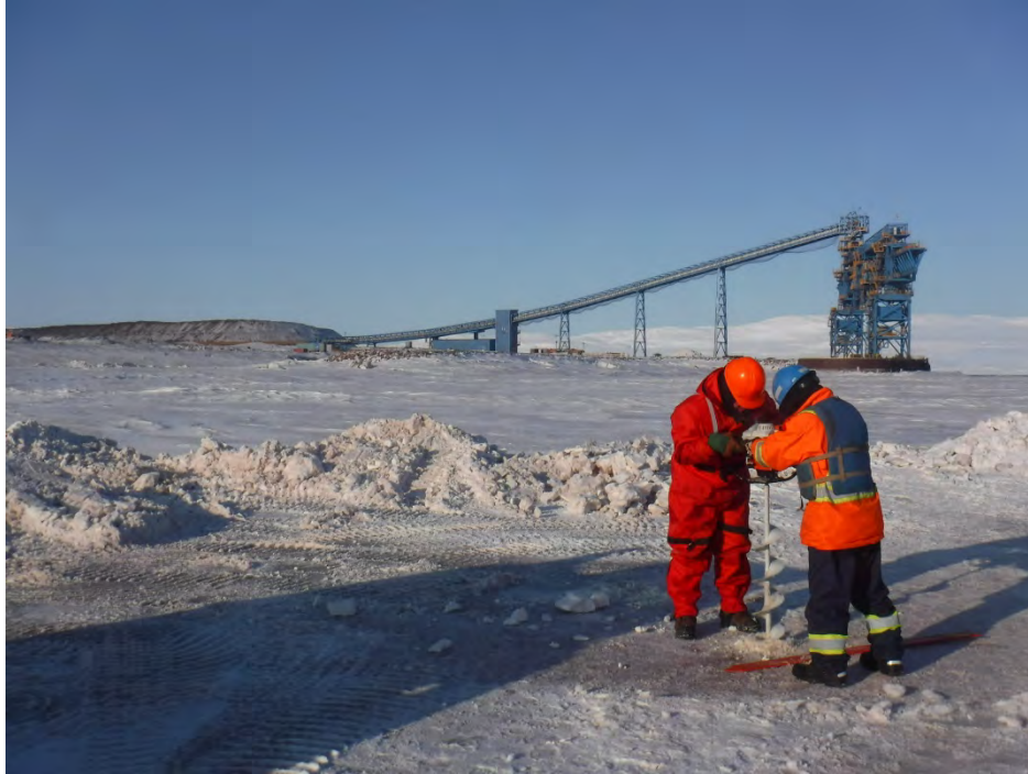
PHOTO 1 - Post-Drilling Conditions at CPT-01B, April 2018
