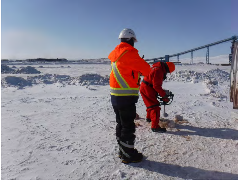
PHOTO 3 - Post-Drilling Conditions at CPT-05, April 2018
