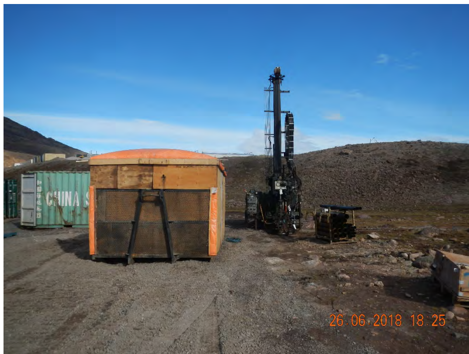
PHOTO 2 - Drilling Conditions at BH18-TF-8N, June 2018
