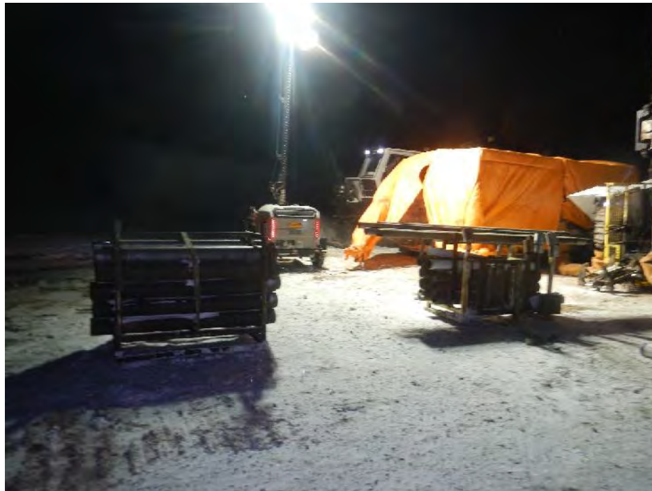
PHOTO 2 - Drilling Conditions at BH18-M001, April 2018
