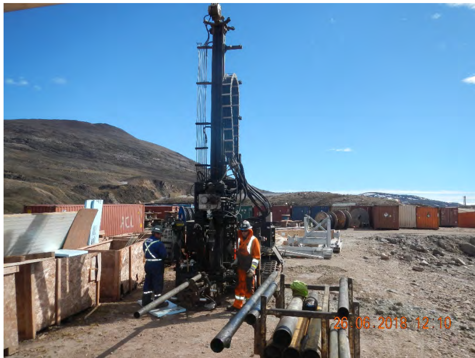
PHOTO 2 - Drilling Conditions at BH18-TF-7N, June 2018
