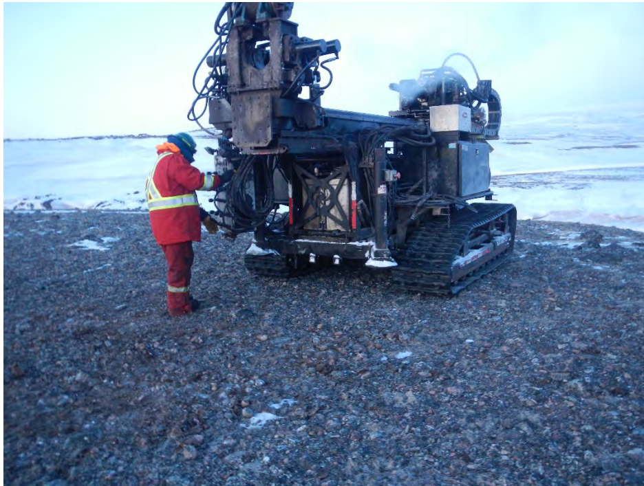
PHOTO 1 - Pre-Drilling Conditions at BH18-BR102-2, April 2018
