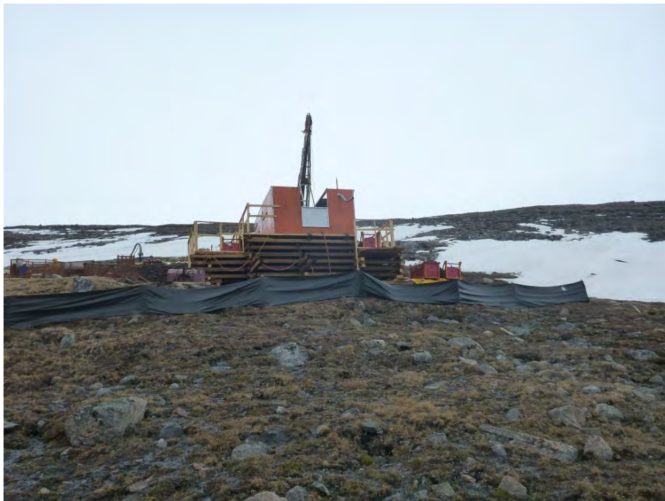
PHOTO 2 - Drilling Conditions at MR3-18-239, June 2018
