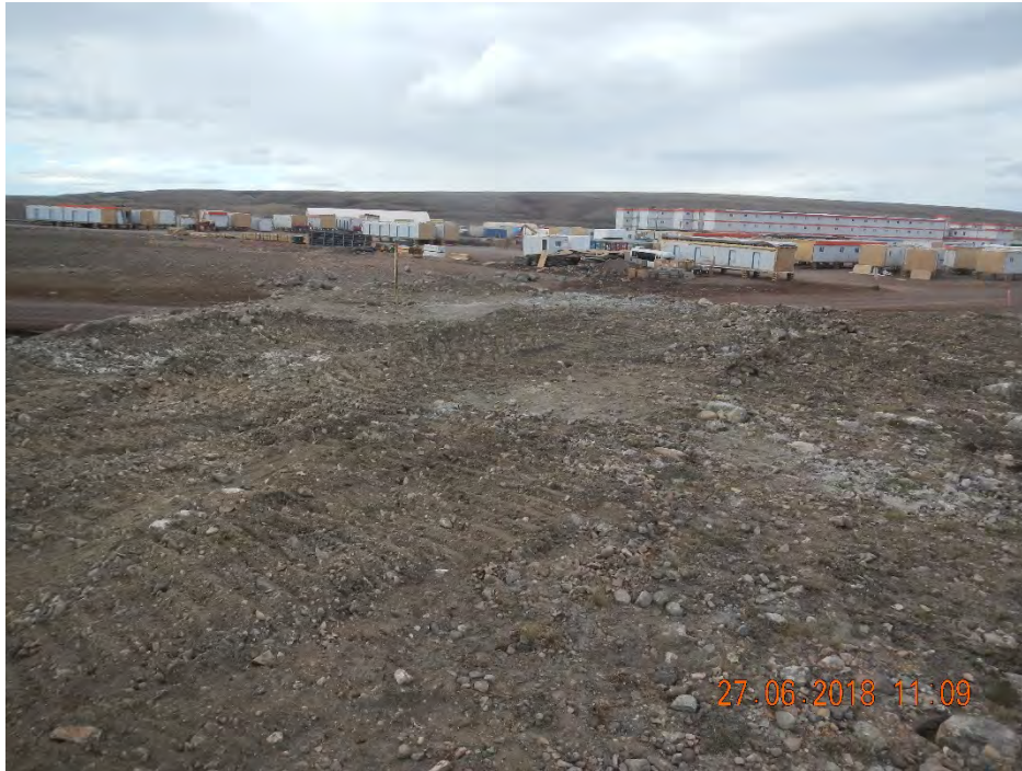
PHOTO 3 - Post-Drilling Conditions at BH18-TF-02, June 2018
