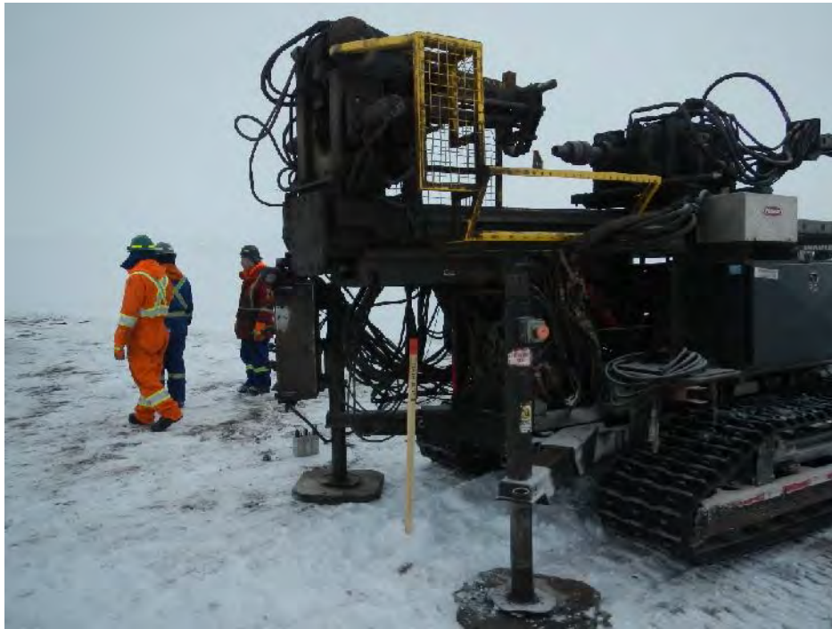
PHOTO 1 - Pre-Drilling Conditions at BH18-M002, April 2018
