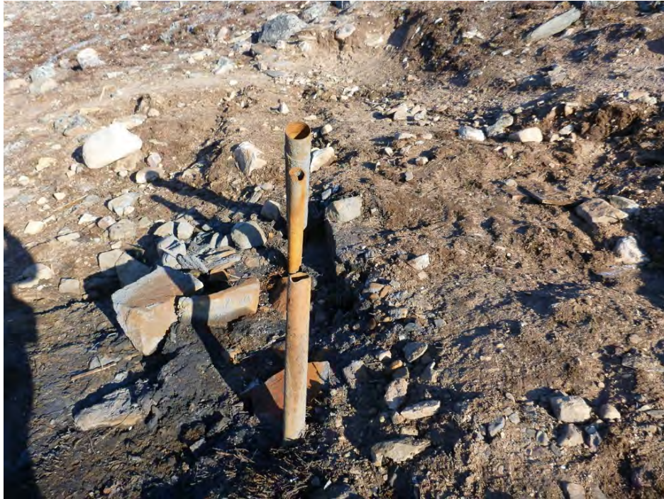
PHOTO 3 - Post-Drilling Conditions at MR2-18-242, June 2018
