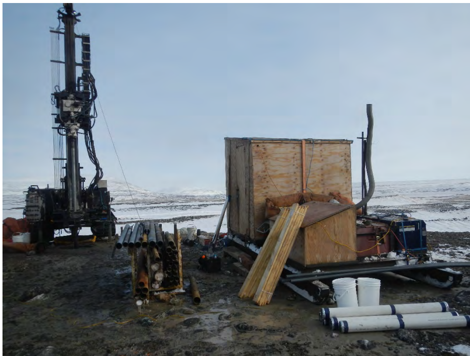
PHOTO 2 - Drilling Conditions at BH18-BR102-2, April 2018
