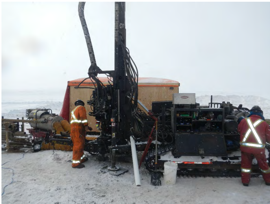
PHOTO 2 - Drilling Conditions at BH18-BR70-1, April 2018
