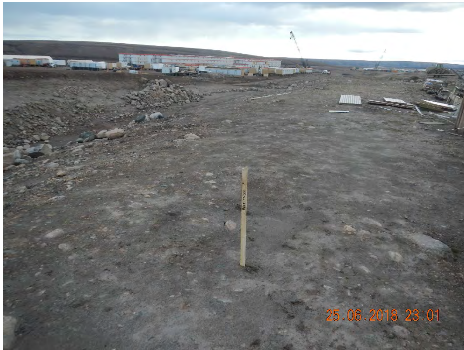
PHOTO 1 - Pre-Drilling Conditions at BH18-TF-7N, June 2018
