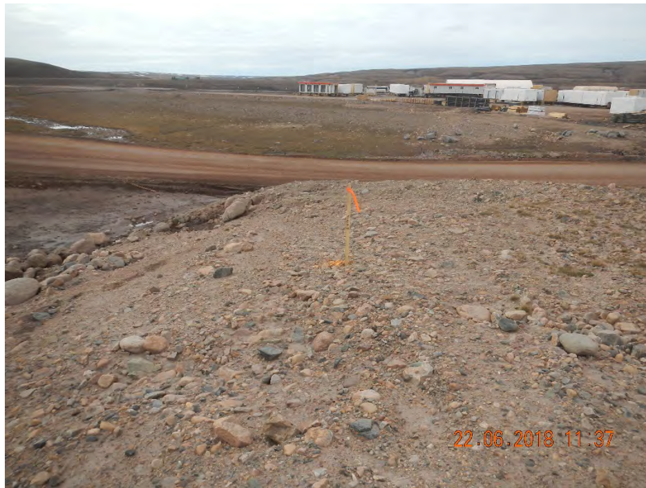
PHOTO 1 - Pre-Drilling Conditions at BH18-TF-02, June 2018
