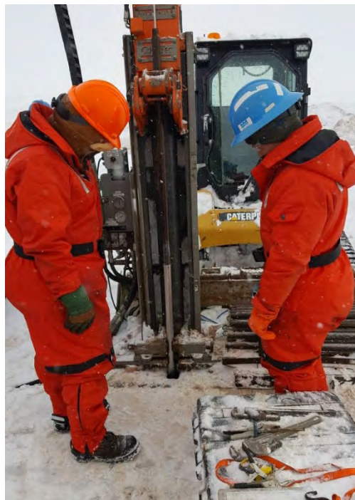
PHOTO 2 - Drilling Conditions at CPT-05, April 2018
