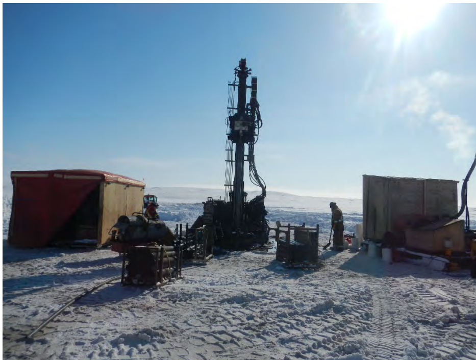
PHOTO 2 - Drilling Conditions at BH18-BR70-2, April 2018
