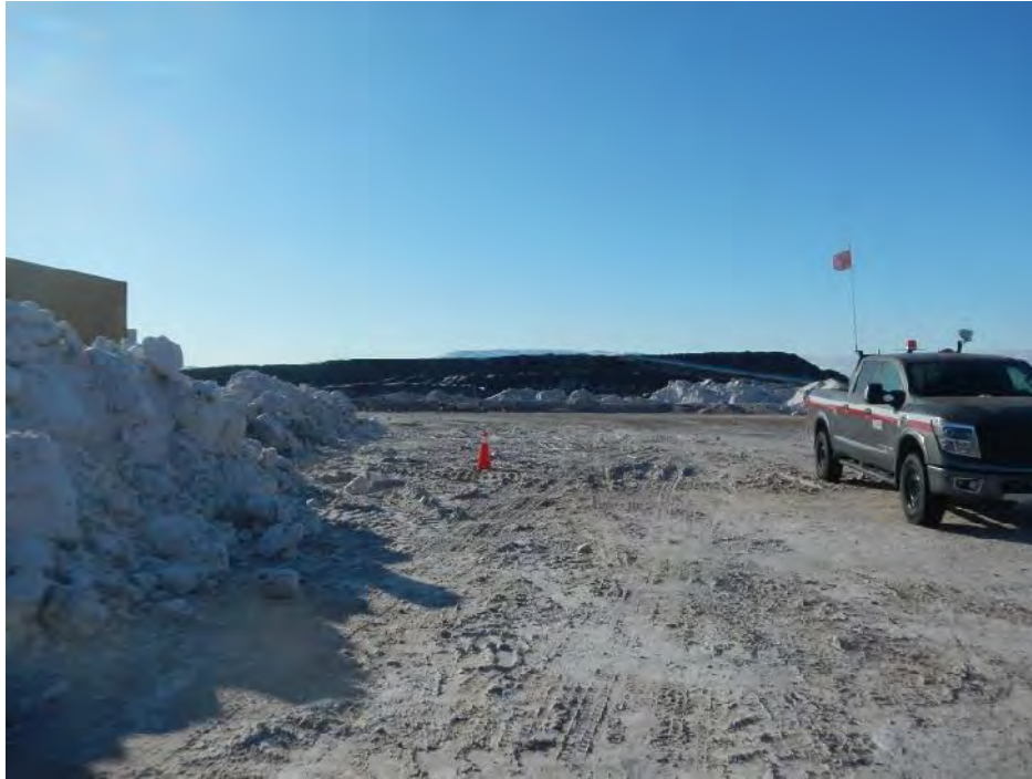
PHOTO 3 - Post-Drilling Conditions at BH18-004, April 2018
