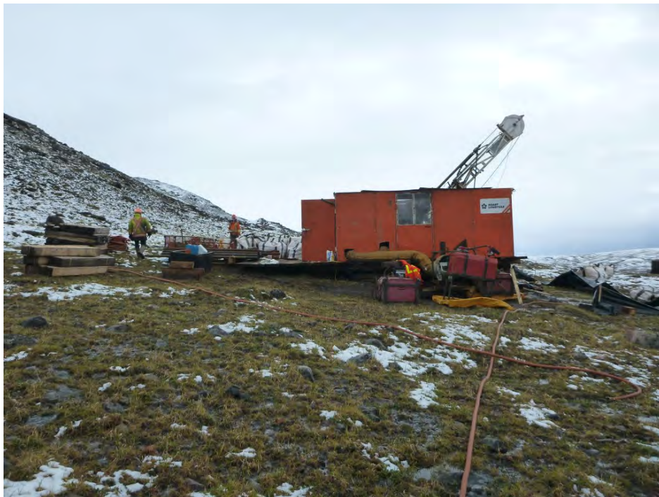
PHOTO 2 - Drilling Conditions at MR2-18-245, July 2018
