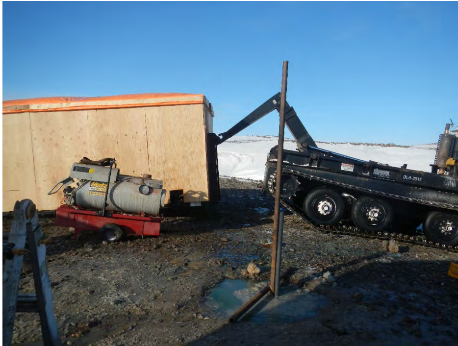
PHOTO 3 - Post-Drilling Conditions at BH18-BR102-2, April 2018
