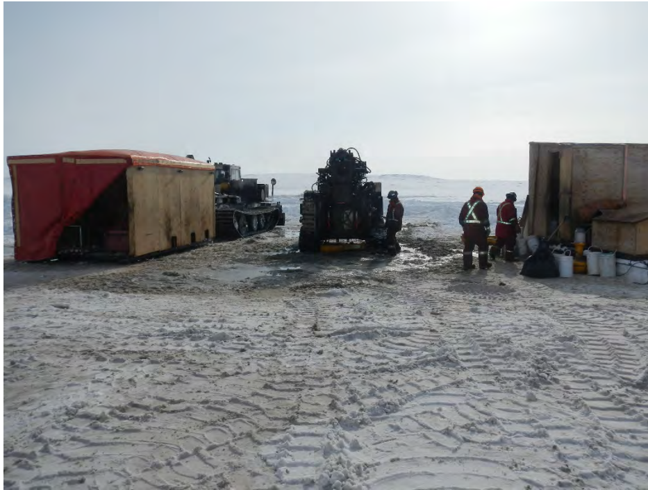
PHOTO 3 - Post-Drilling Conditions at BH18-BR70-2, April 2018
