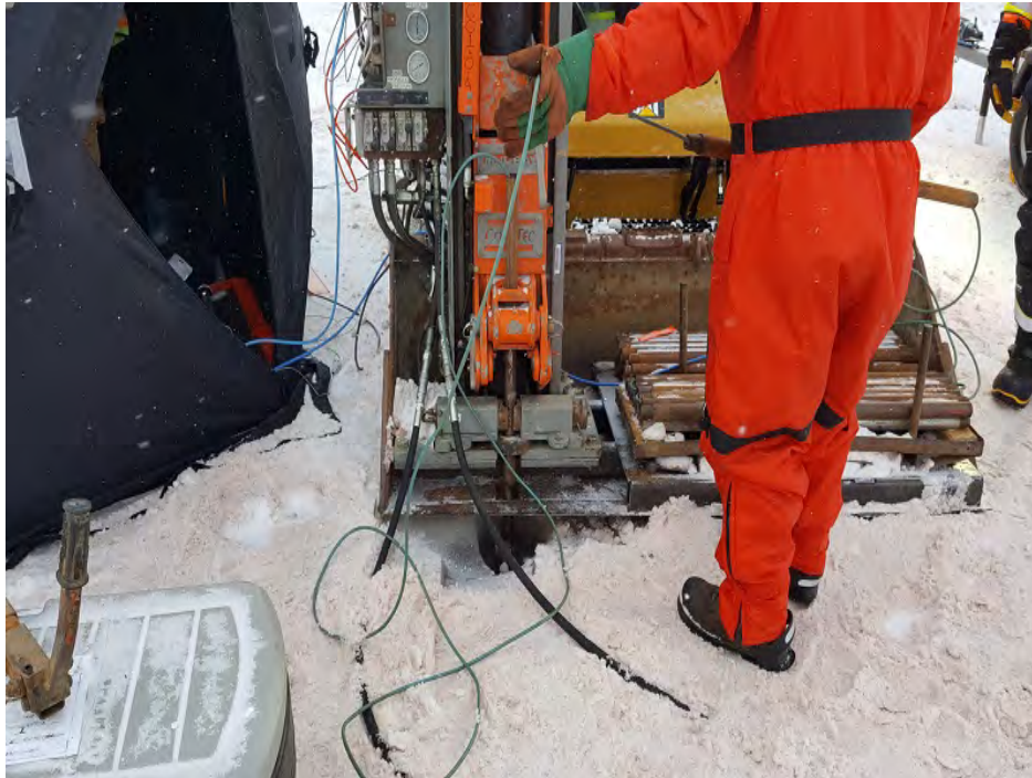
PHOTO 1 - Drilling Conditions at CPT-08, April 2018
