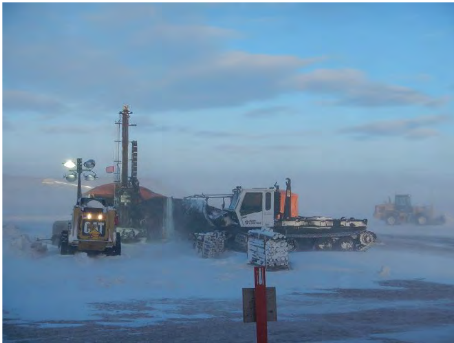
PHOTO 2 - Drilling Conditions at BH18-004, April 2018
