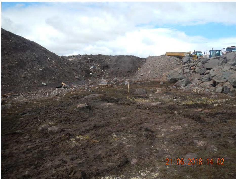
PHOTO 2 - Post-Drilling Conditions at BH18-TW-02, June 2018
