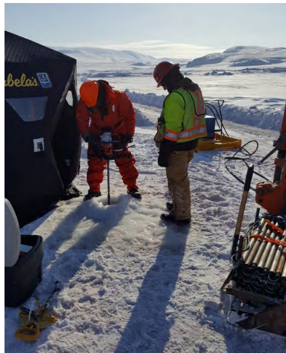
PHOTO 2 - Drilling Conditions at CPT-03, April 2018
