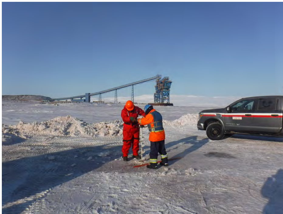
PHOTO 2 - Post-Drilling Conditions at CPT-01, April 2018
