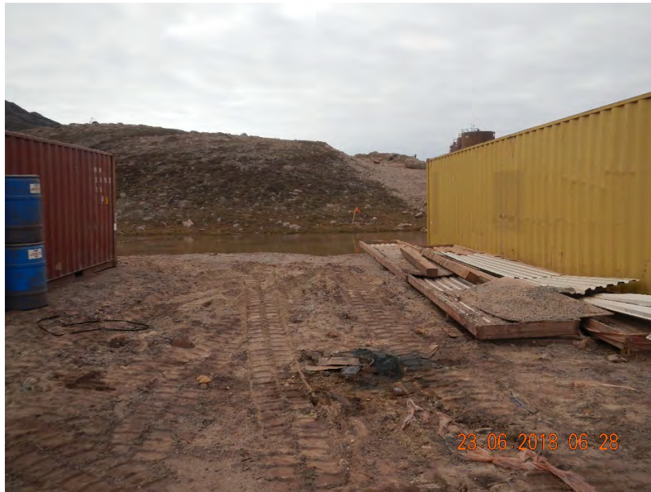
PHOTO 1 - Pre-Drilling Conditions at BH18-TF-01, June 2018
