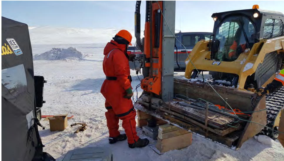
PHOTO 1 - Drilling Conditions at CPT-02, April 2018
