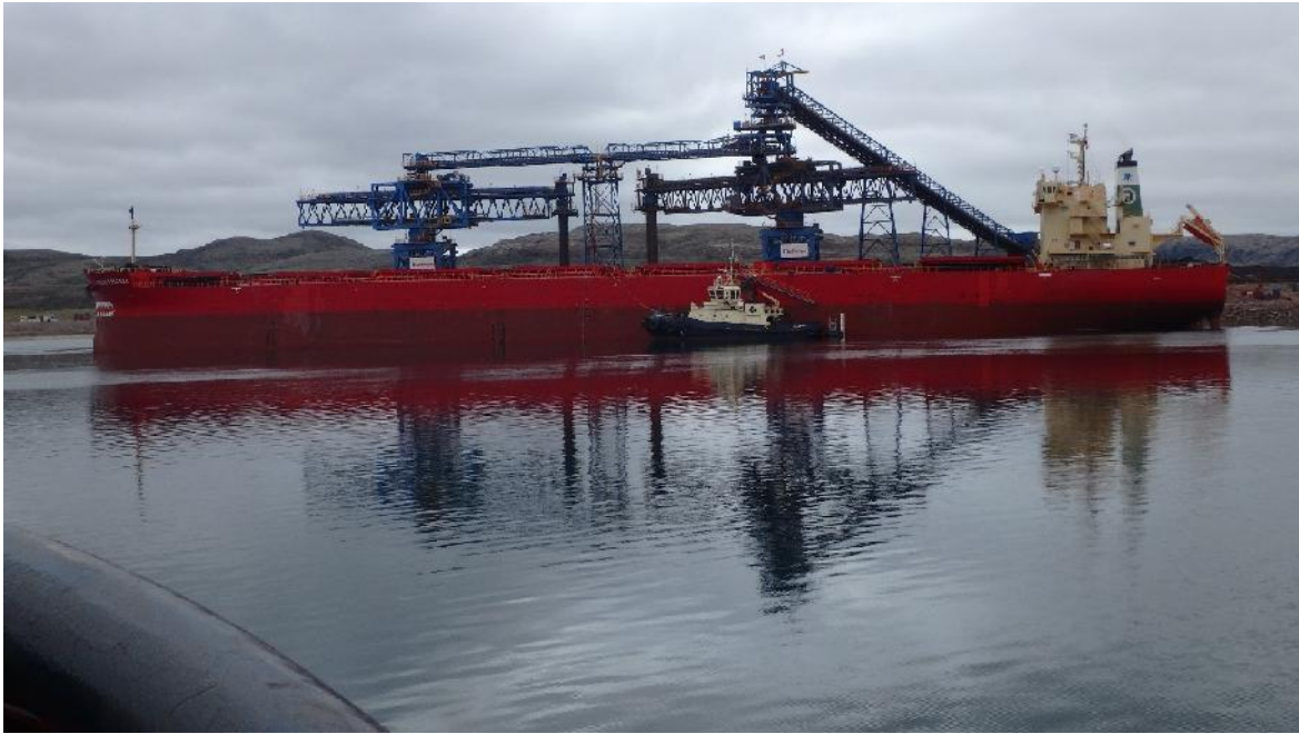
PHOTO 5 - Milne Port Ship loader with Ore freighter berthed at Ore Dock, 2016
