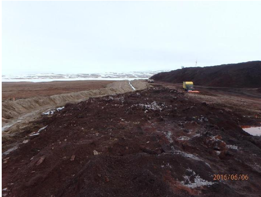
Figure 10: View looking North showing Drainage Ditch Diversion around Frozen Ore/Snow Stockpile
