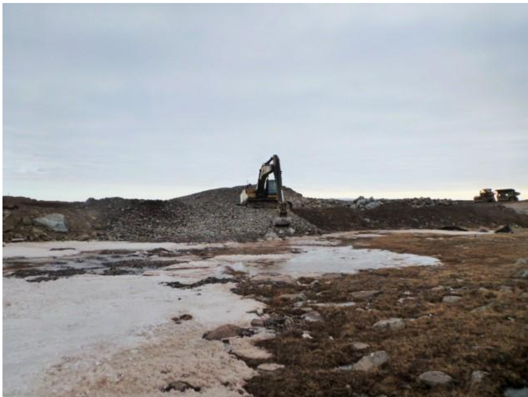
PHOTO 4 – Excavator Armorizing the Mine Haul Road Embankment, May 2016
