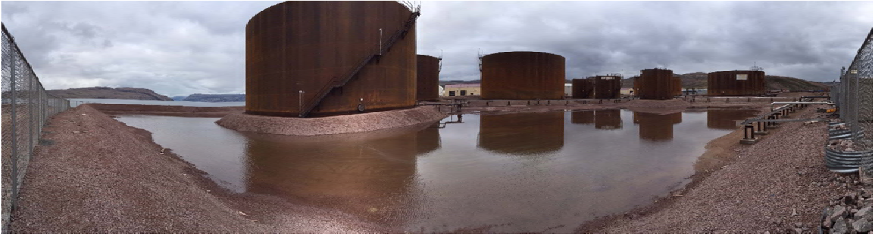
Photograph 3: Showing impacted water pooling within north and west side of interior containment berm. August 8, 2016
