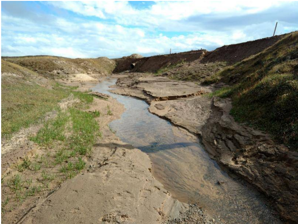
Photo 6 – BG -31 flowing clear downstream of culvert on July 31, 2016
