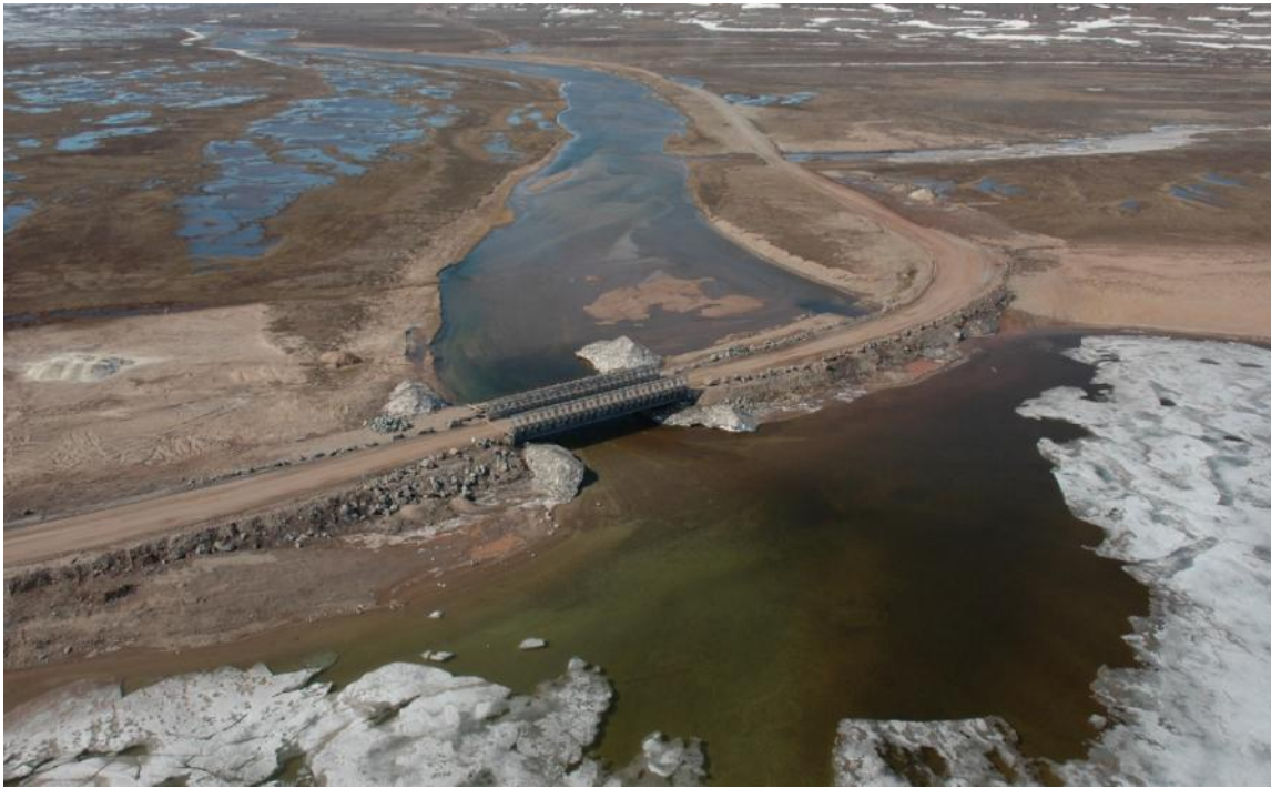
PHOTO 5 – Aerial view of the Milne Port Tote Road Km 17 Bridge, June 2016
