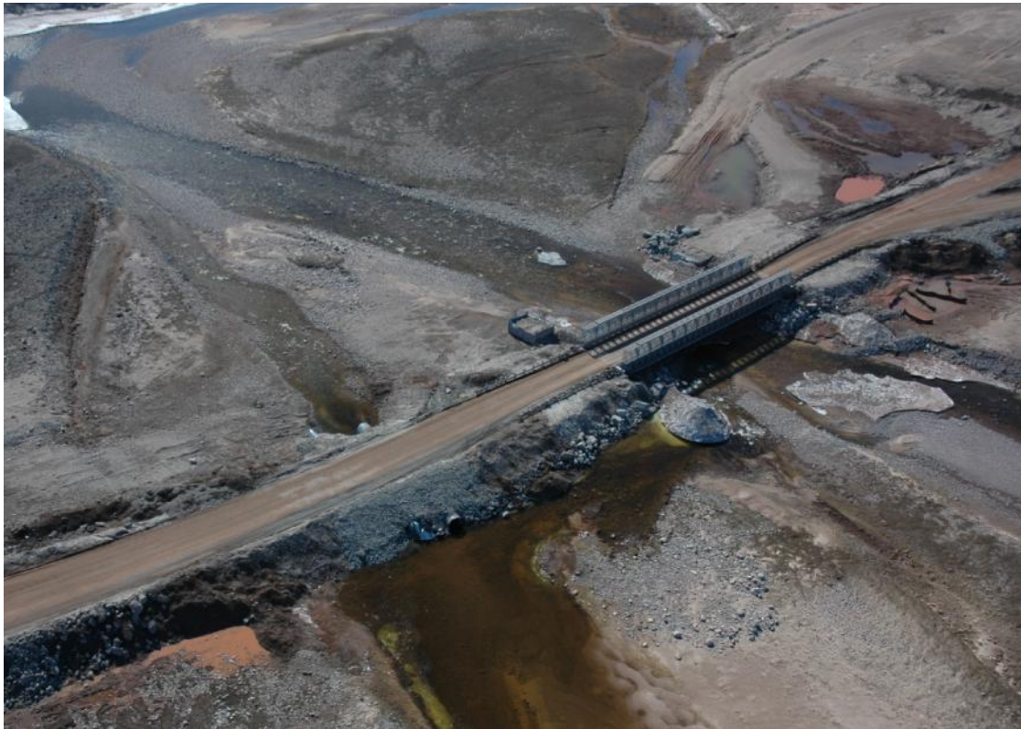
PHOTO 6 – Aerial view of the Milne Port Tote Road Km 97 Bridge, June 2016
