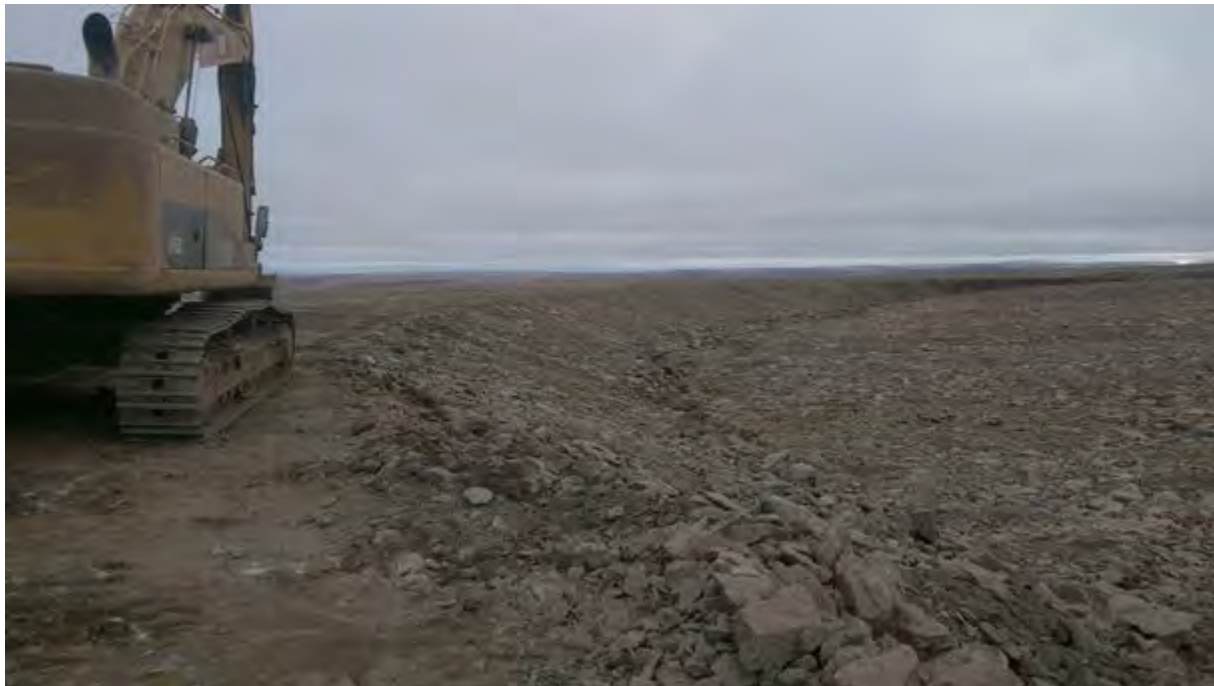
Figure 3: Berm after Fill Placement
