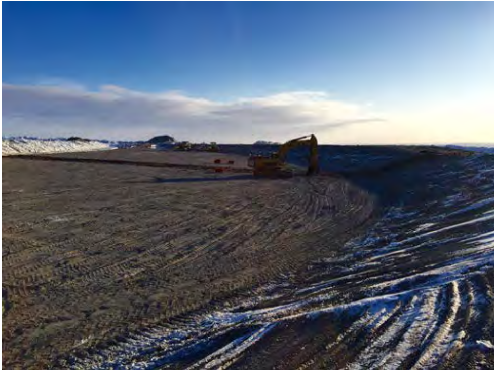
Figure 4: Liner Installation Started
