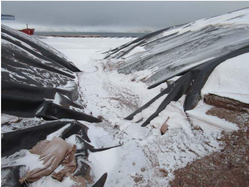
East Drainage Pond
