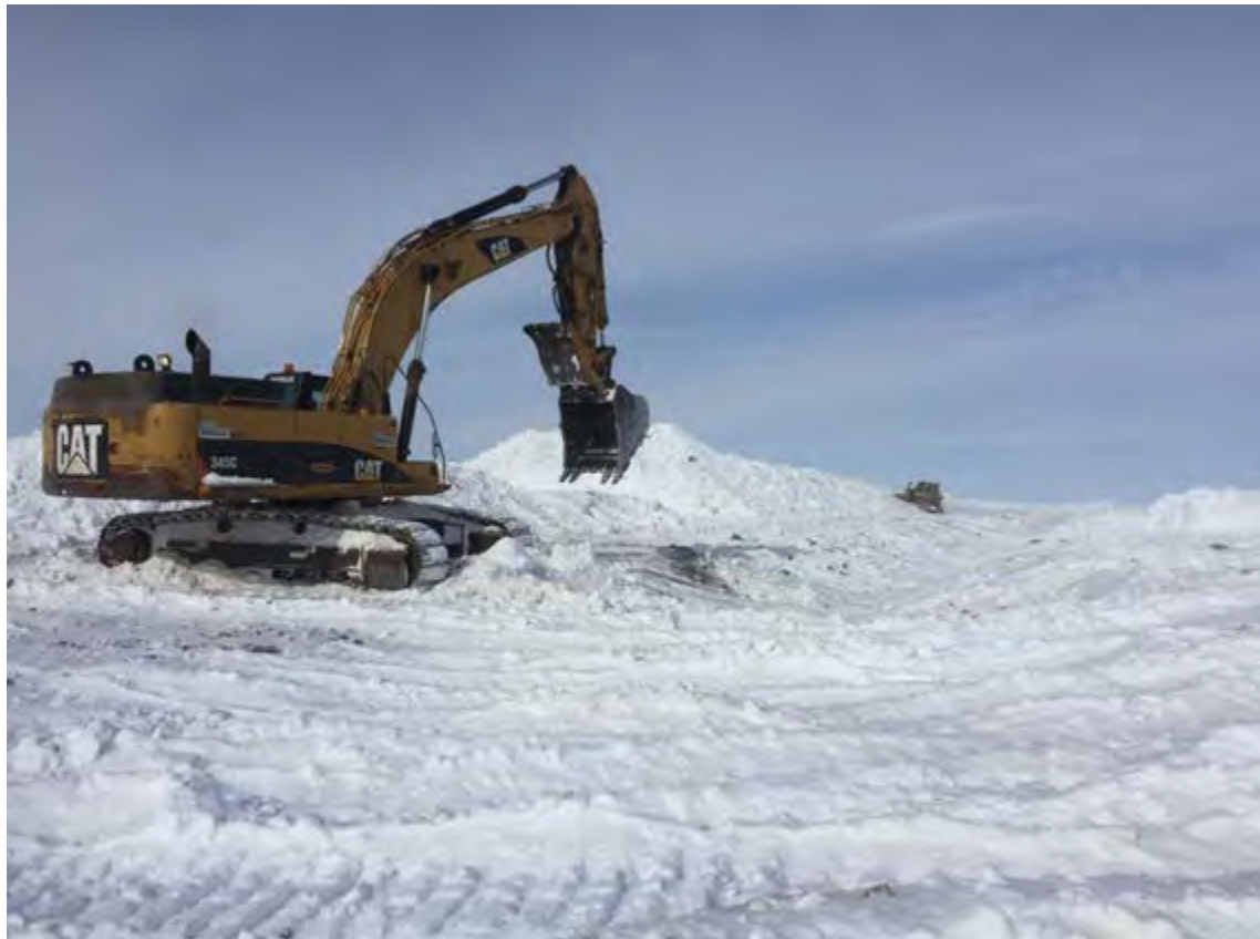
Figure 11: Clearing Snow from Ditch
