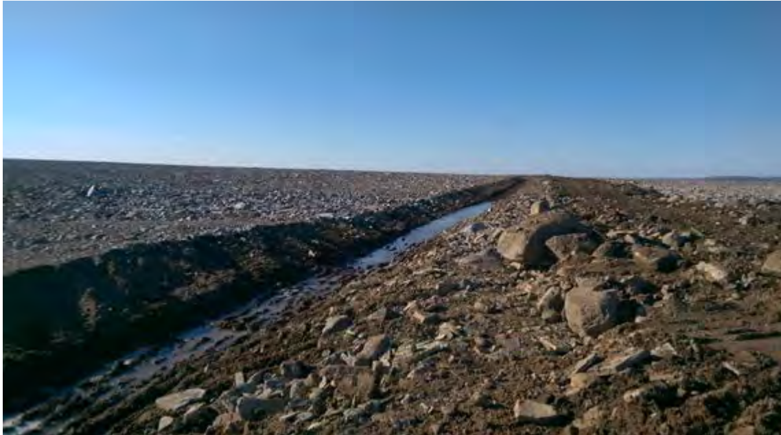
Figure 10: Ditch After Excavation
