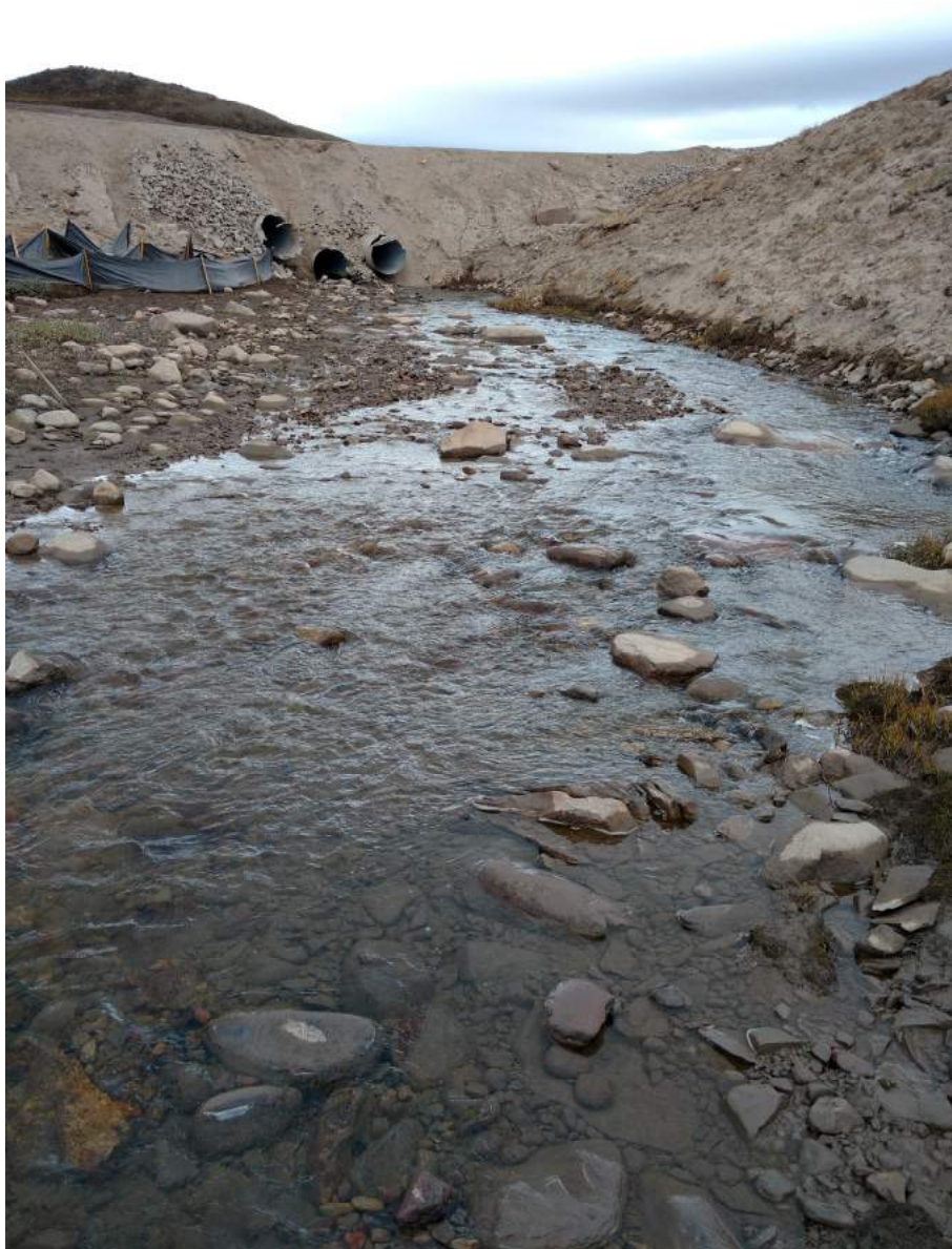
Photo 5 – Water flowing clear downstream of BG-01 (km 100) on August 26, 2016
