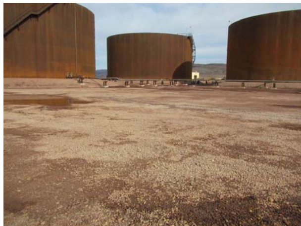
Photograph 5: Showing west side of interior containment berm during collection activities. August 31, 2016
