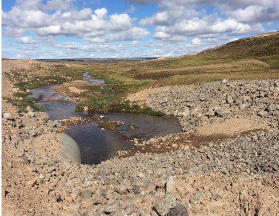
Photo 3 – Clear flow at outlet of BG-17 with armoured banks on July 22, 2016
