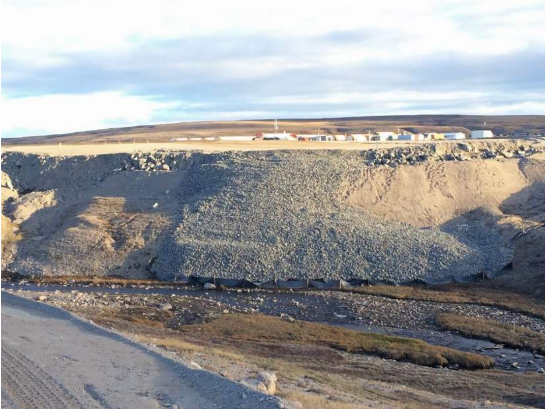
Photo 1 – Current status of stable slope face by Camp Lake Tributary #1 on August 30, 2016.
