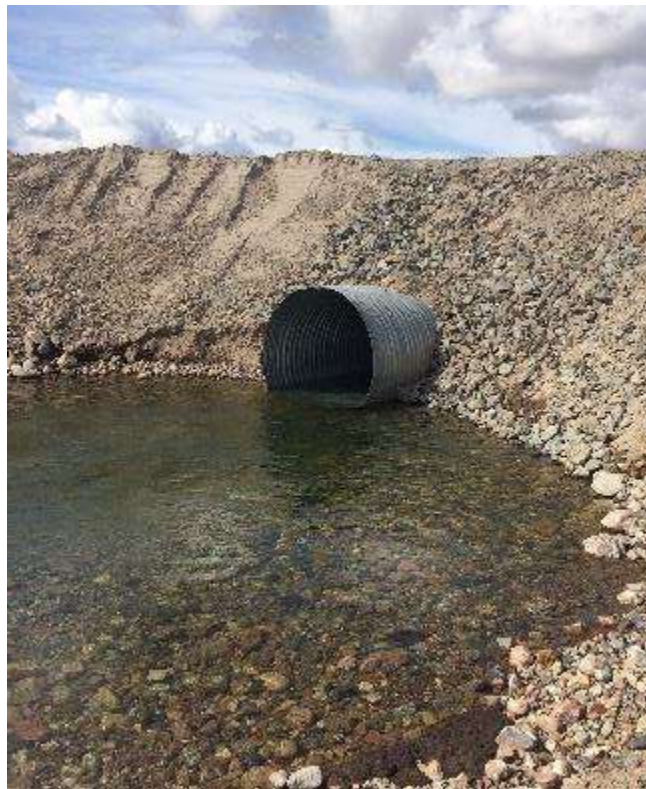
Photo 2 – Outlet of CV223 with armoured slope on July 22, 2016
