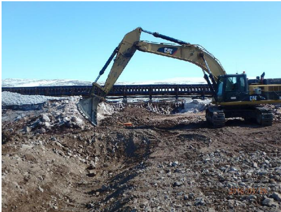
Figure 5: View looking North East with Swale being Excavated
