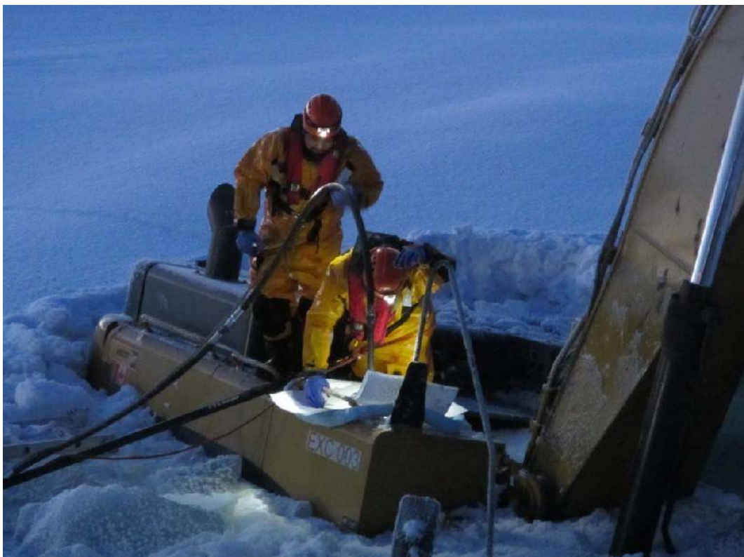
Photo 2 – Diesel Fuel Recovery
