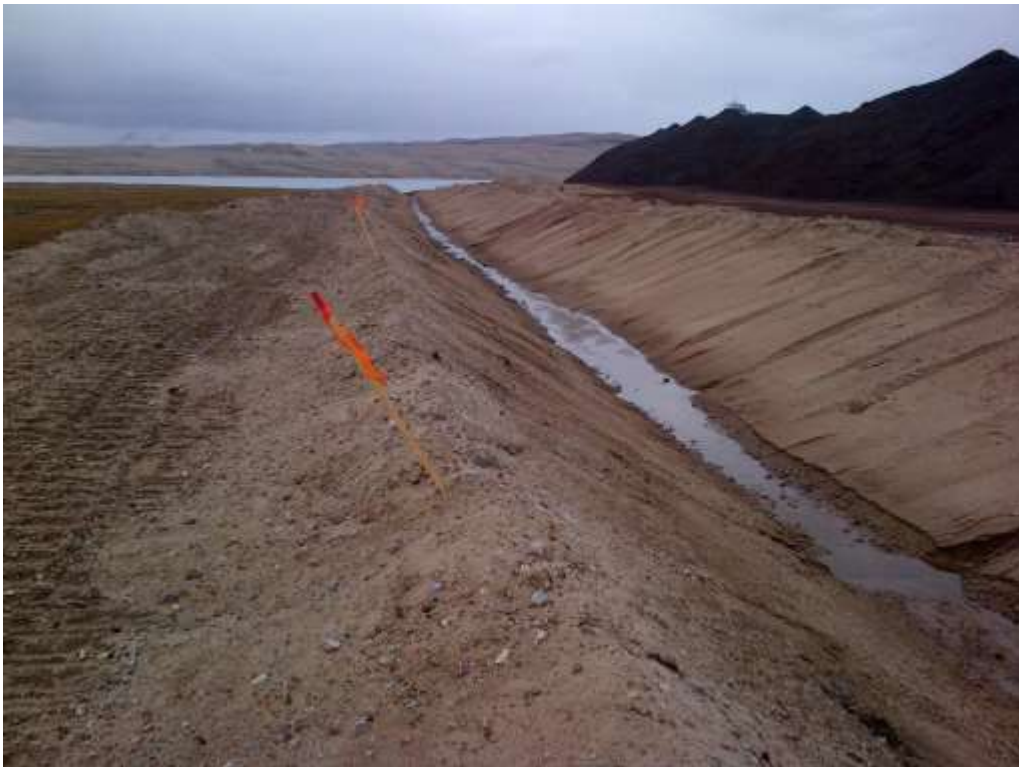
Photo 2 – Completed ditch work at the Milne Port Ore Pad on July 18, 2016
