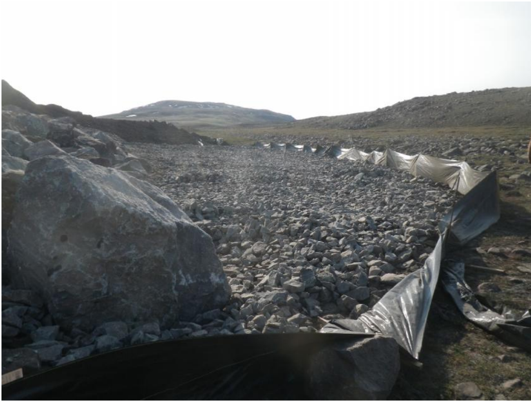
PHOTO 5 – Siltation mitigation measures at the toe of the Crusher Pad, July 2016
