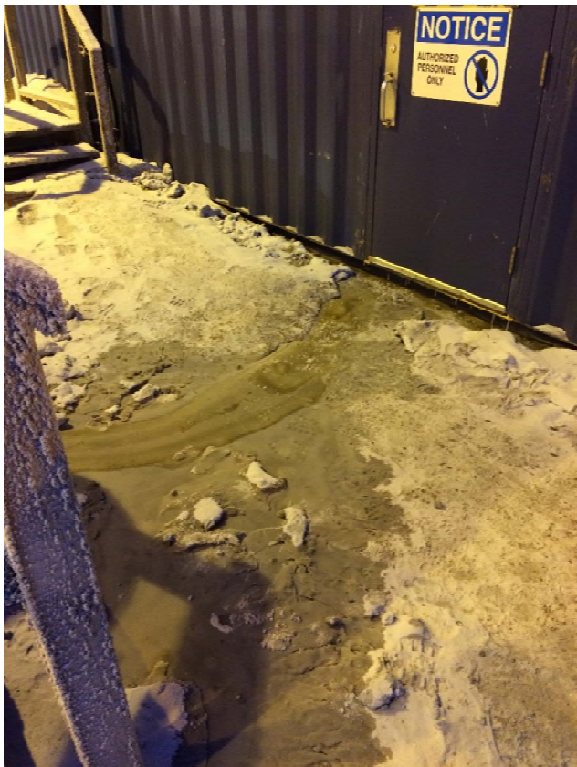
Photo 1 – WWTP Raw Sewage Spill
