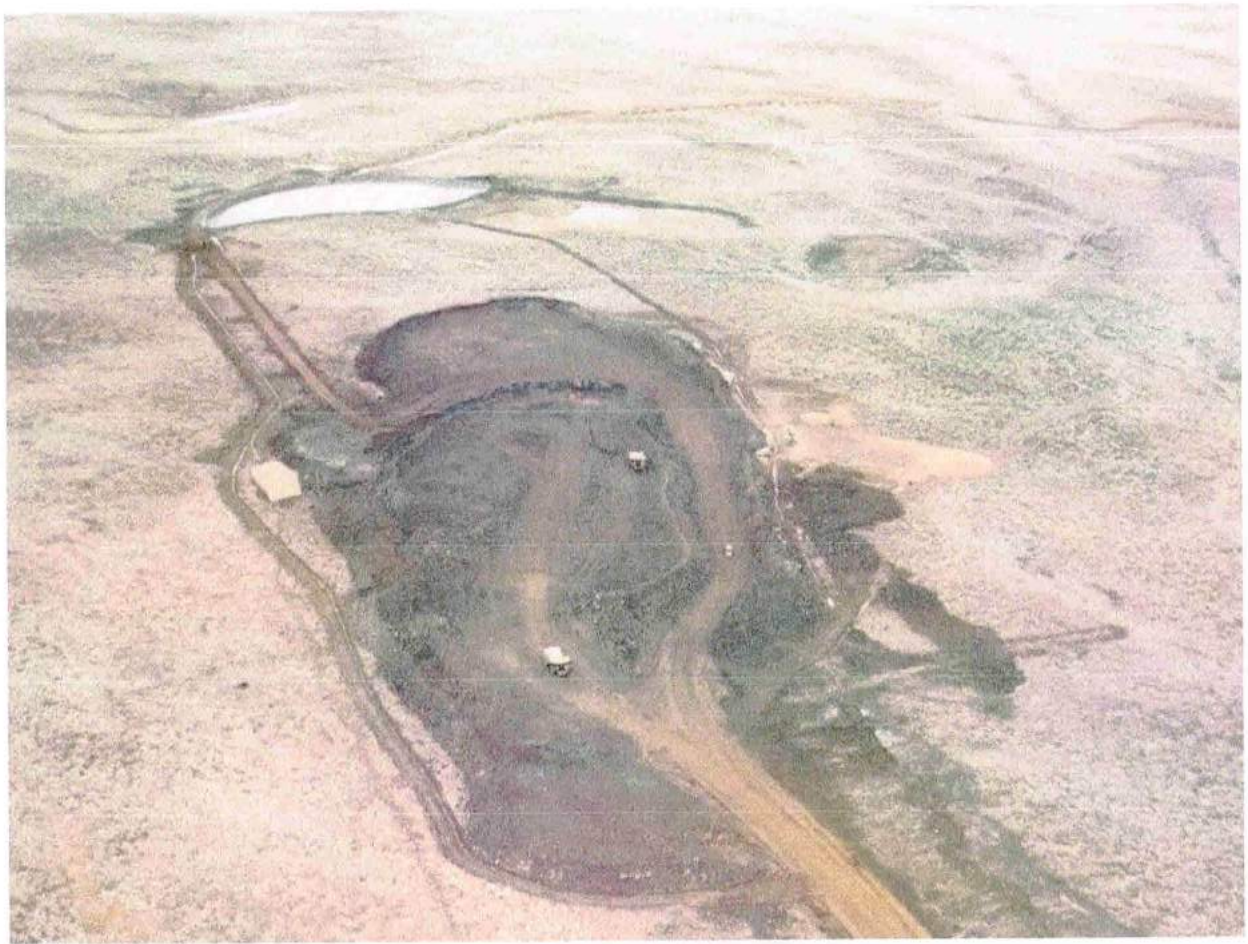
Aerial Photograph Waste Pile Drainage Containment
