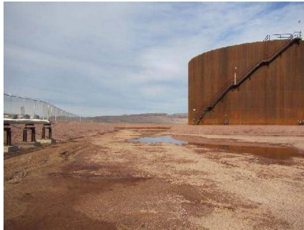
Photograph 4: Showing north side of interior containment berm during collection activities. August 31, 2016
