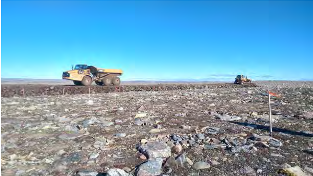
Figure 2: Fill Placement for Berm Construction
