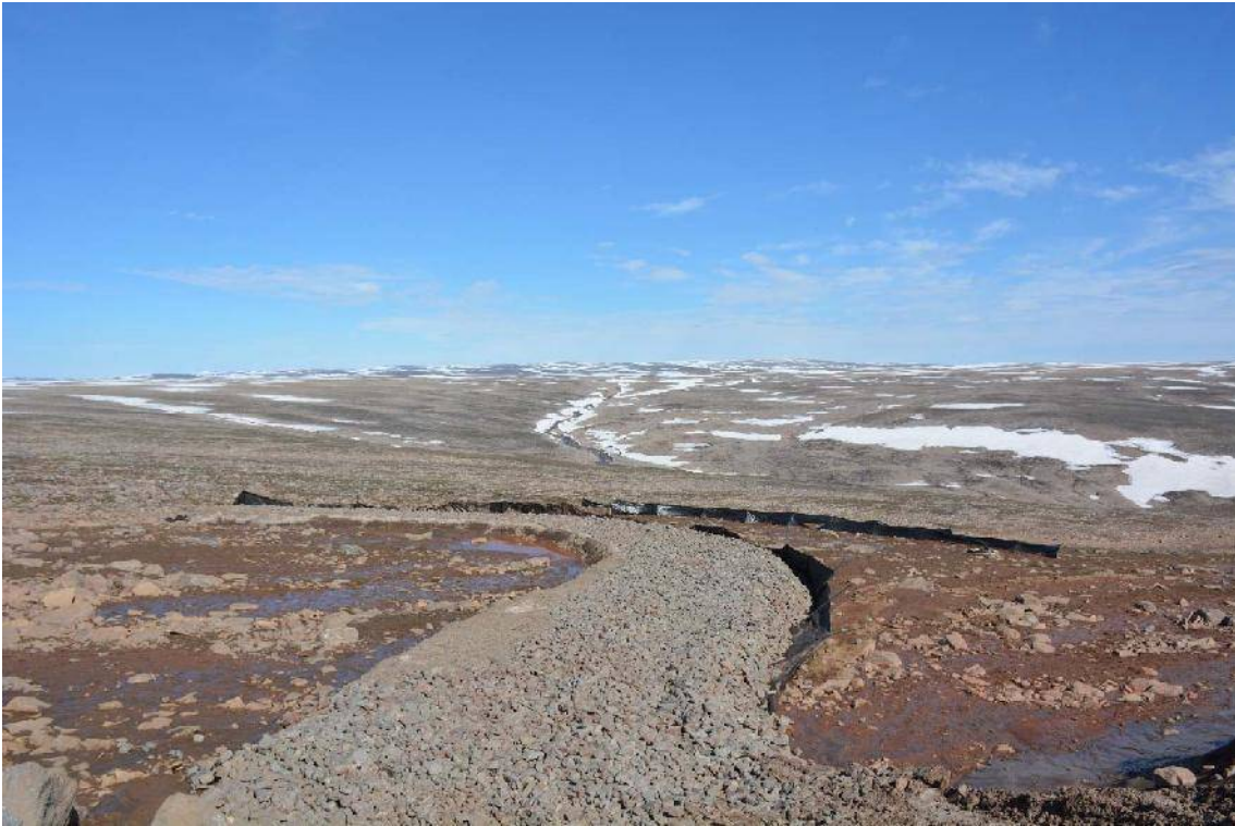
Photo 1– Checkdam #5 constructed at Km 108.5. Picture taken on July 5, 2016.
