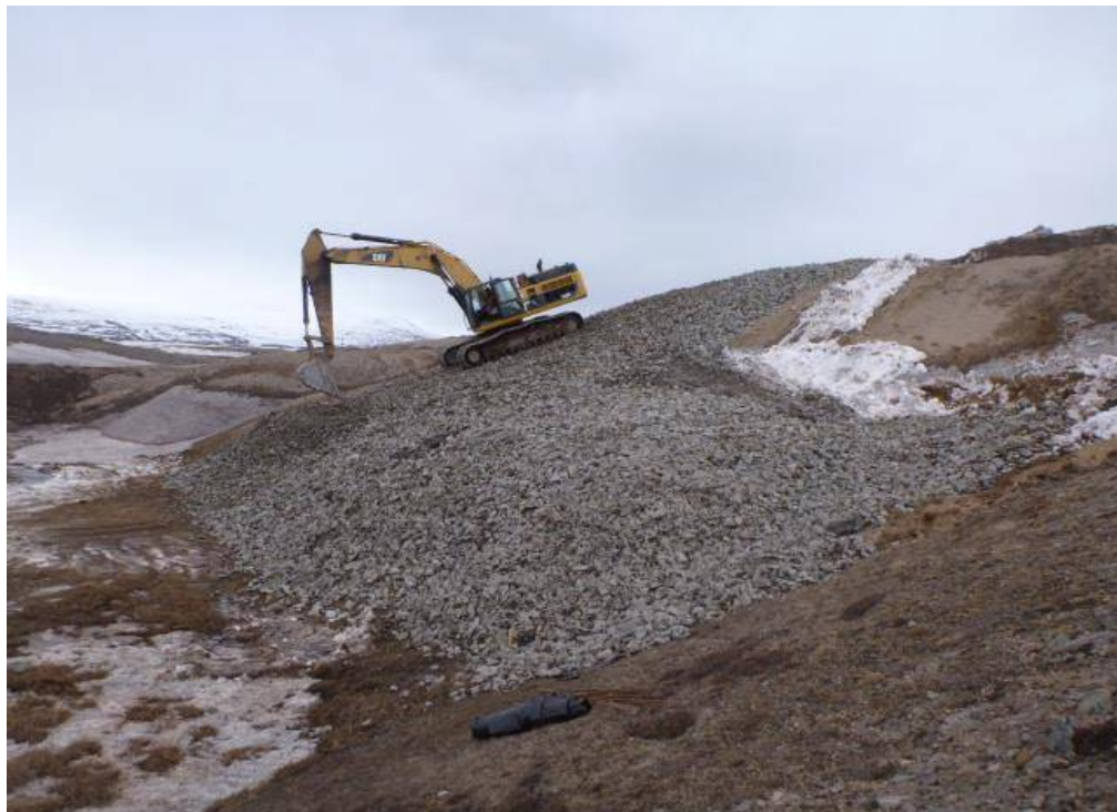
Photo 4 – June 4 th 2016. Slumping stream bank reinforced with 6" aggregate.
