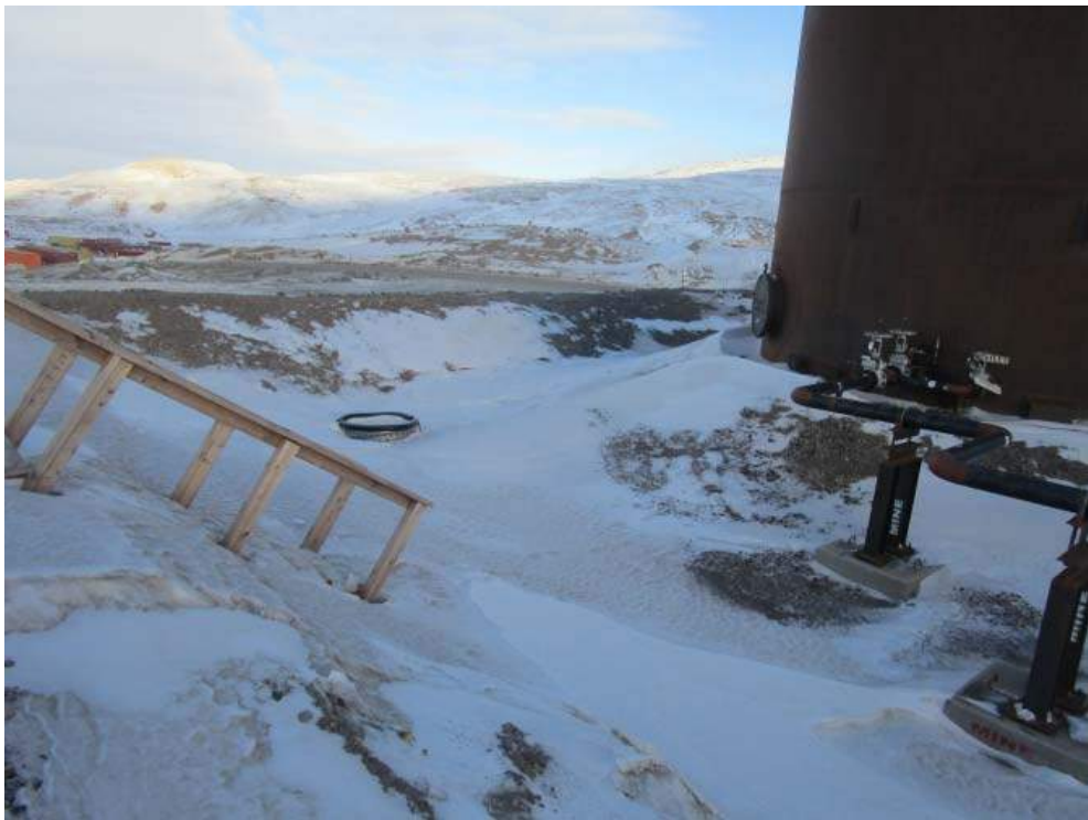
Bulk Fuel Storage – Sump Installed
