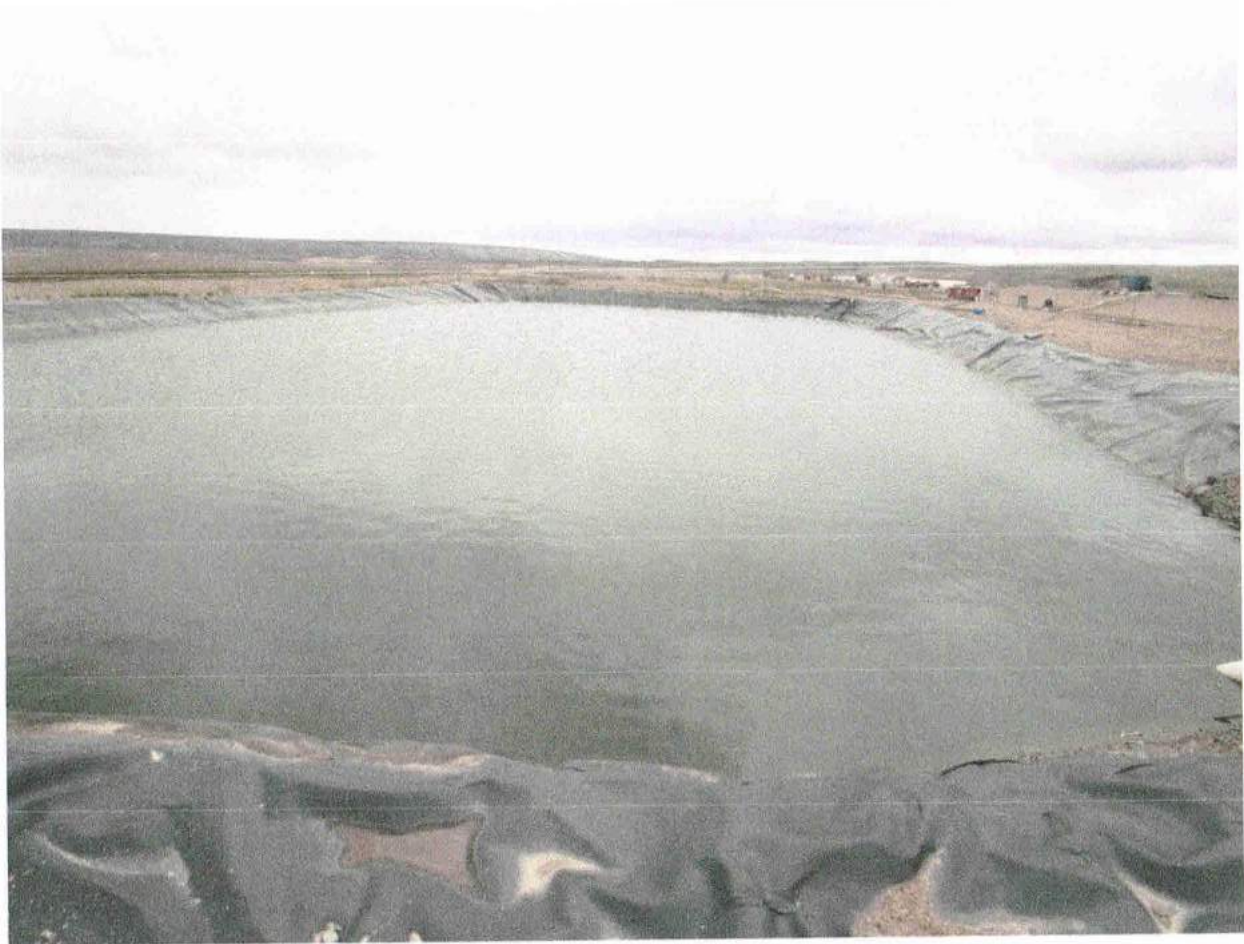
Polishing Waste Stabilization Pond #3.
