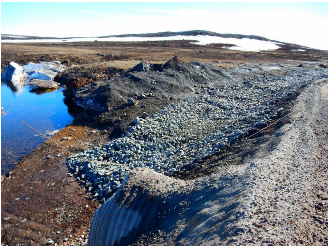
PHOTO 8 – Armoring and Ditch Repair, KM 94 Culvert BG04, June 2016
