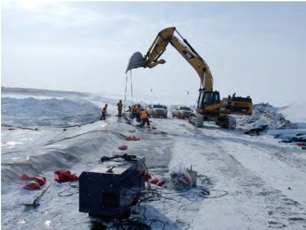
Figure 5: Liner Placement
