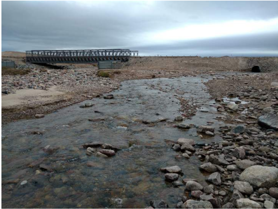
Photo 1 – Water flowing clear downstream of CV223 (km 97) on August 26, 2016
