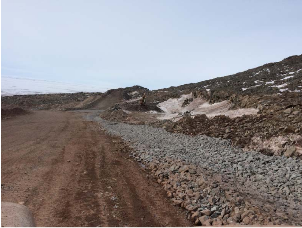
Mine Haul Road Ditching and Riprapping Photos – April 2016
