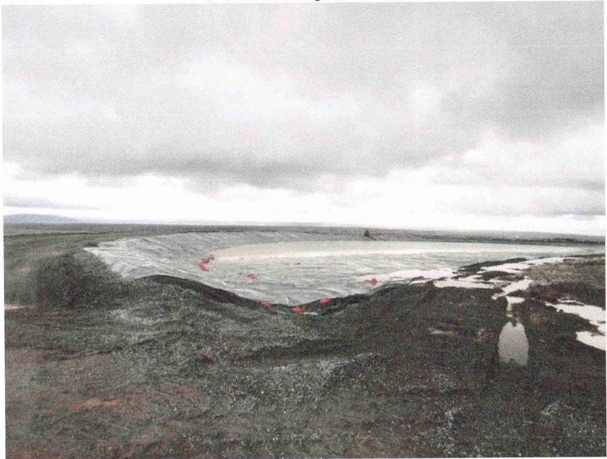
Waste Pile Drainage Containment
