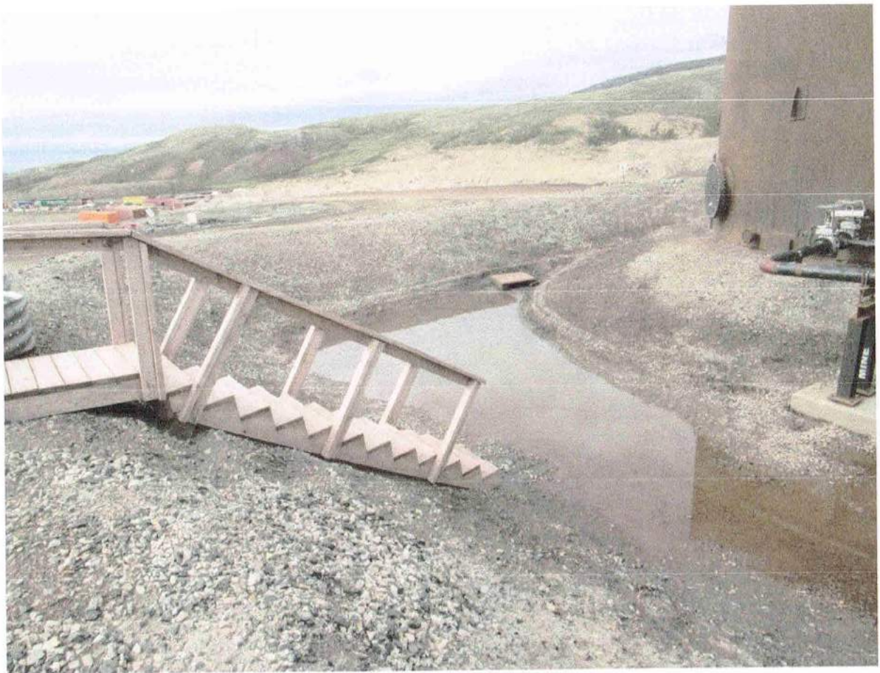
Minesite Steel Fuel Tank Containment
