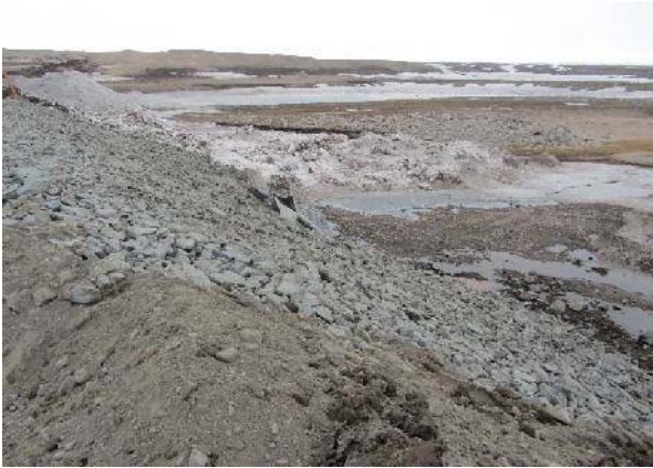
Constructed Drainage Controls Partially Implemented or Completed.
