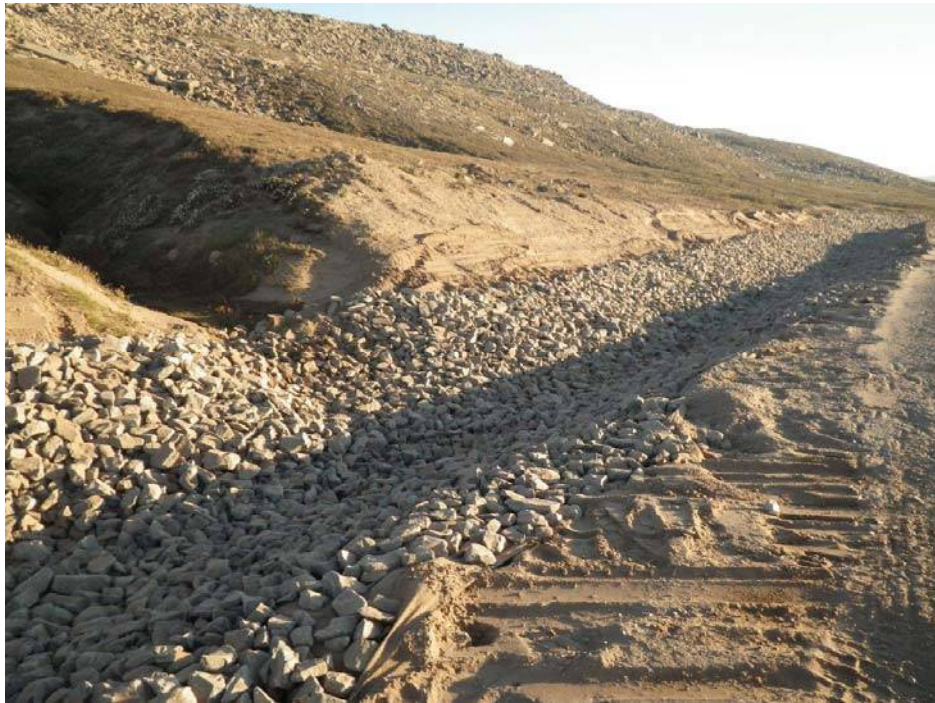
Photo 4- Rip rap in ditch at Km 85
