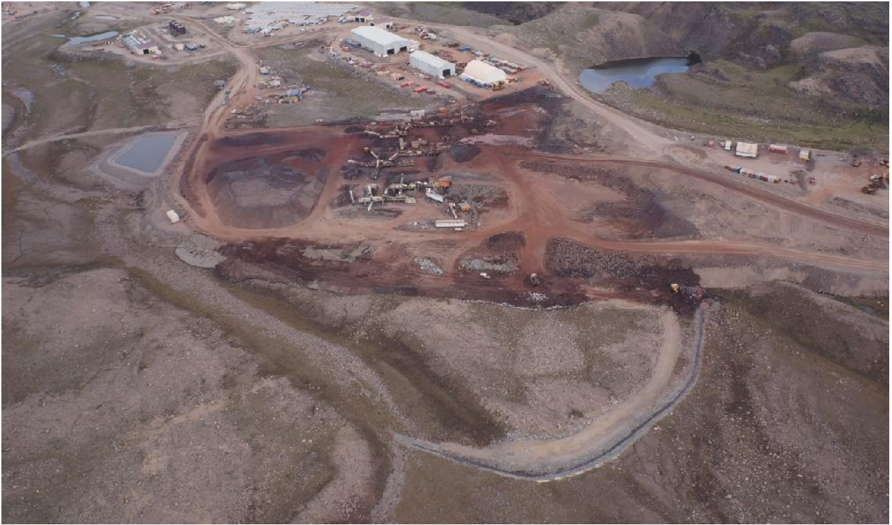
PHOTO 7 - Mary River Mine Site Crusher Pad Ore Stockpile and, Engineered Drainage Ditch and Sedimentation Pond, July 2016
