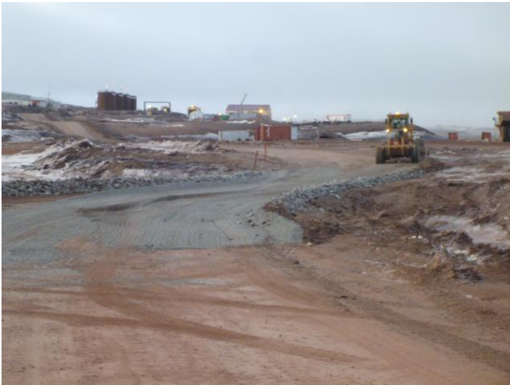
PHOTO 2 – Grading and Capping of CV-186 in Mary River, May, 2016
