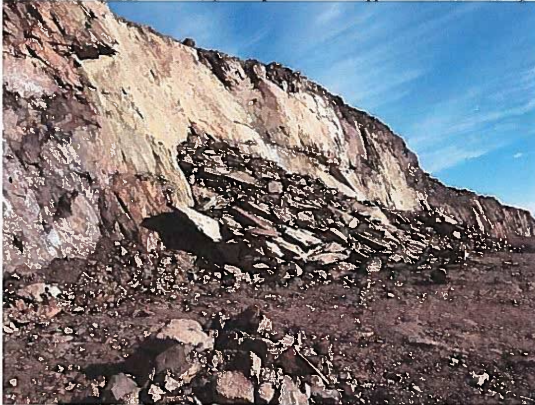
Photo 2: Ongoing raveling from 12m high final pit wall face on upper bench. Ultimate will be ~22m
