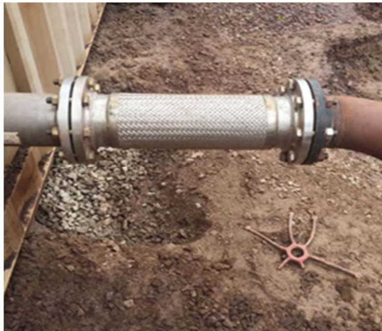
Photograph 2: Section of Braided Flex Pipe after replacement.
