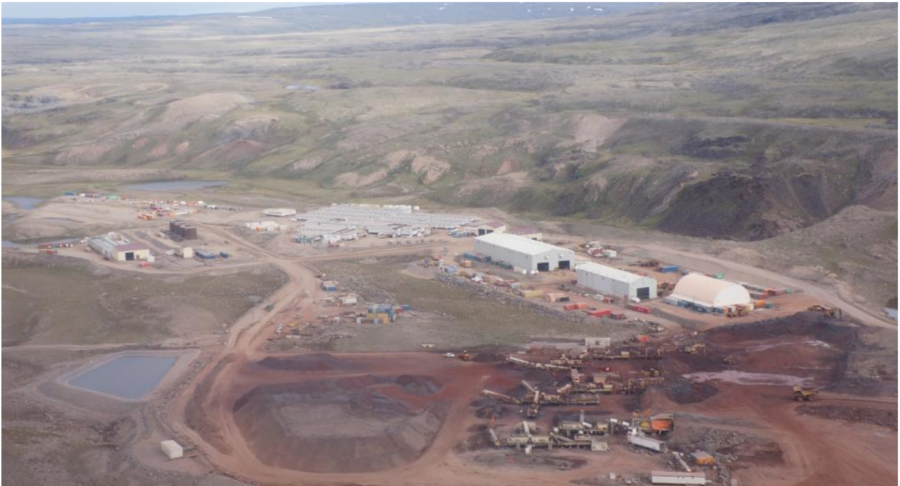
PHOTO 8 - Mary River Mine Site Accommodations Complex, Crusher and Maintenance Yard, July 2016
