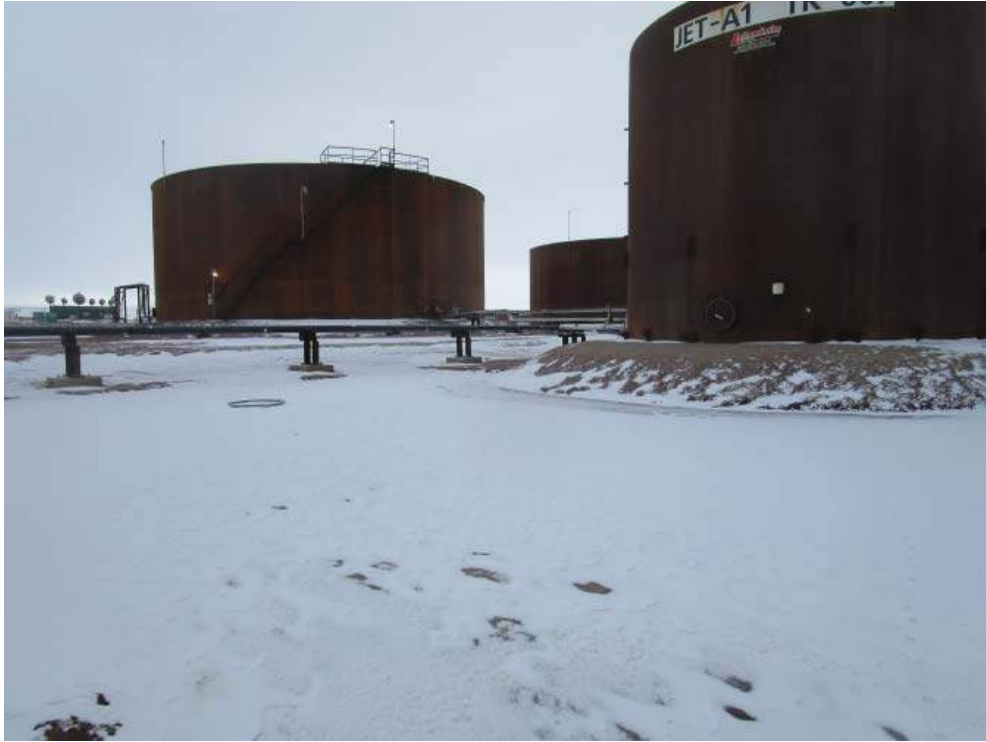
Fuel Tank Farm
