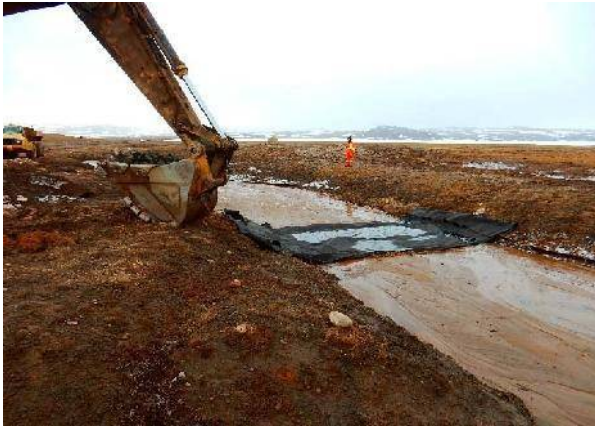
Constructed Drainage Controls Partially Implemented or Completed.
