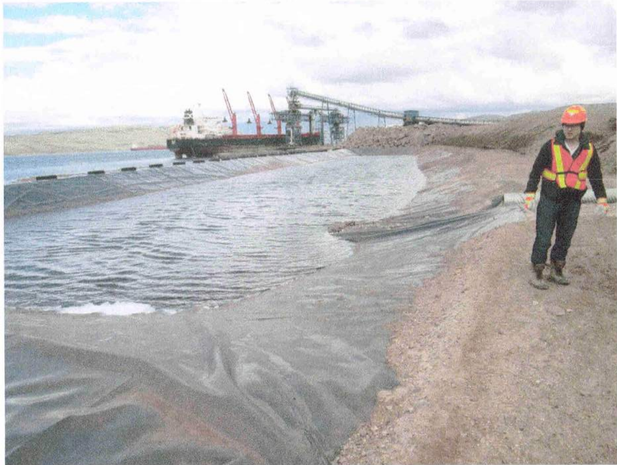
Sediment Pond West
