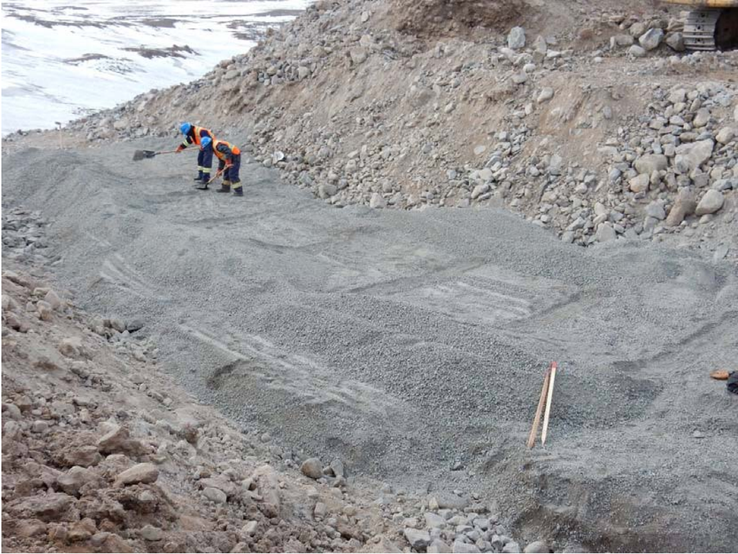
Culvert CV-1 Construction and Installation Photos – May 2016
