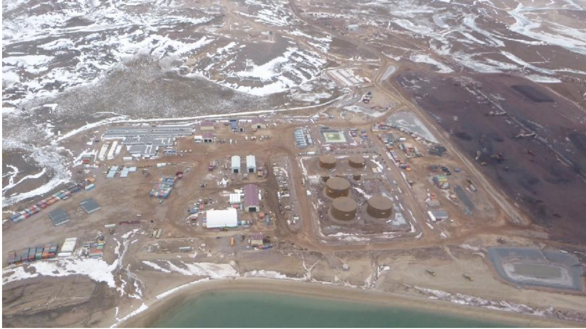
Photo 1 - Milne Port infrastructure, September 2016
