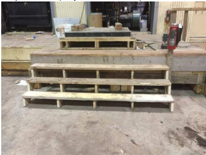
Stairs repaired at the Incinerator Building (Mine Site)
