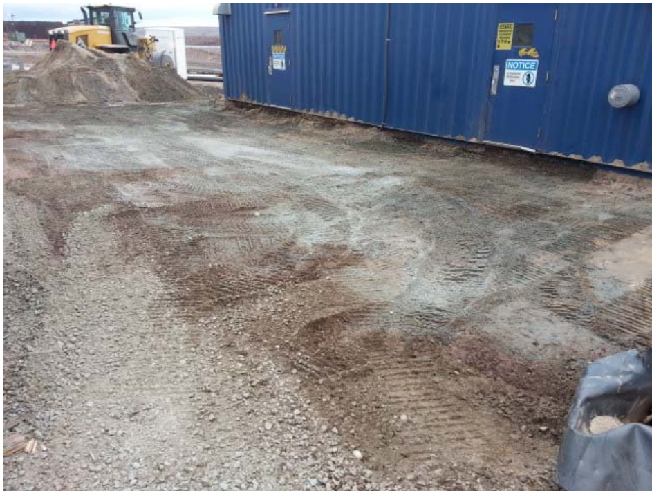
Photo 2. Spill area after removal of contaminated material September 6 th 2016.
