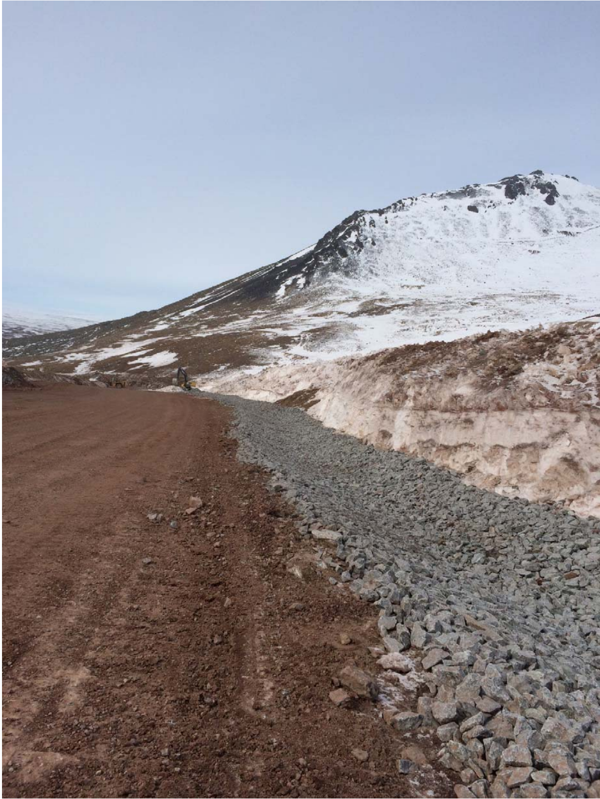
Mine Haul Road Ditching and Riprapping Photos – April 2016
