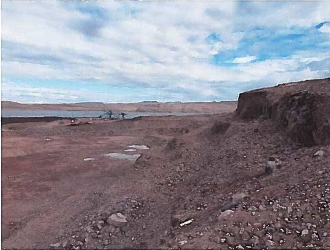
Photo 7: Milne Quarry. Much loose present of faces and bench width less than 8m
