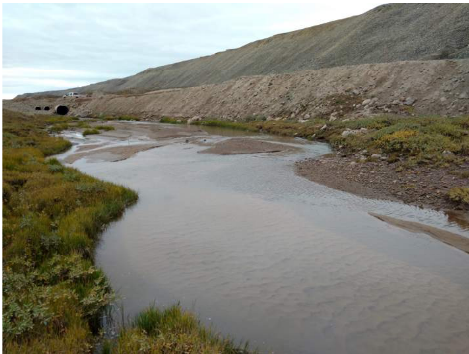
Photo 2 – Water flowing clear downstream of BG-17 (km 90) on August 26, 2016
