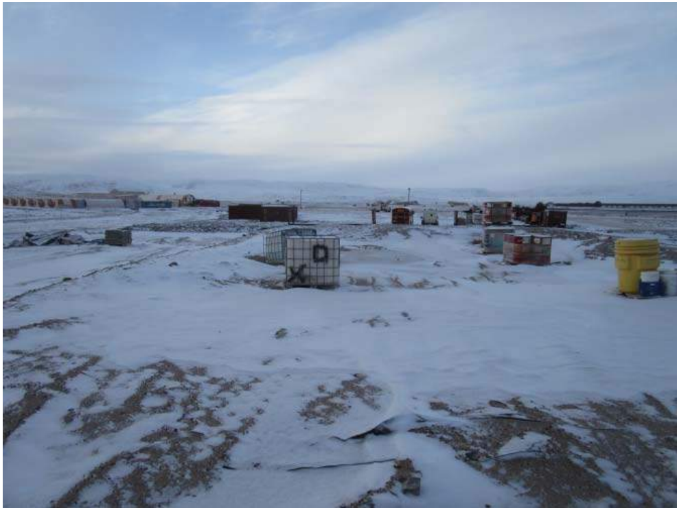
Hazardous Waste Storage MP-HWB-5
