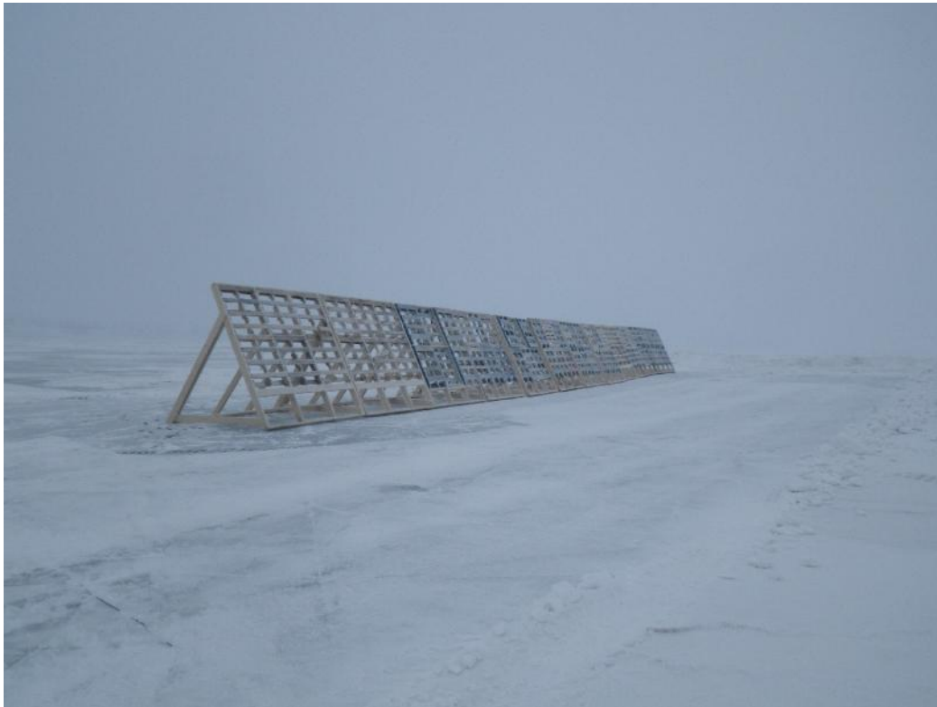
PHOTO 12 – Snow Fence Snow Drift Trial, March 2016
