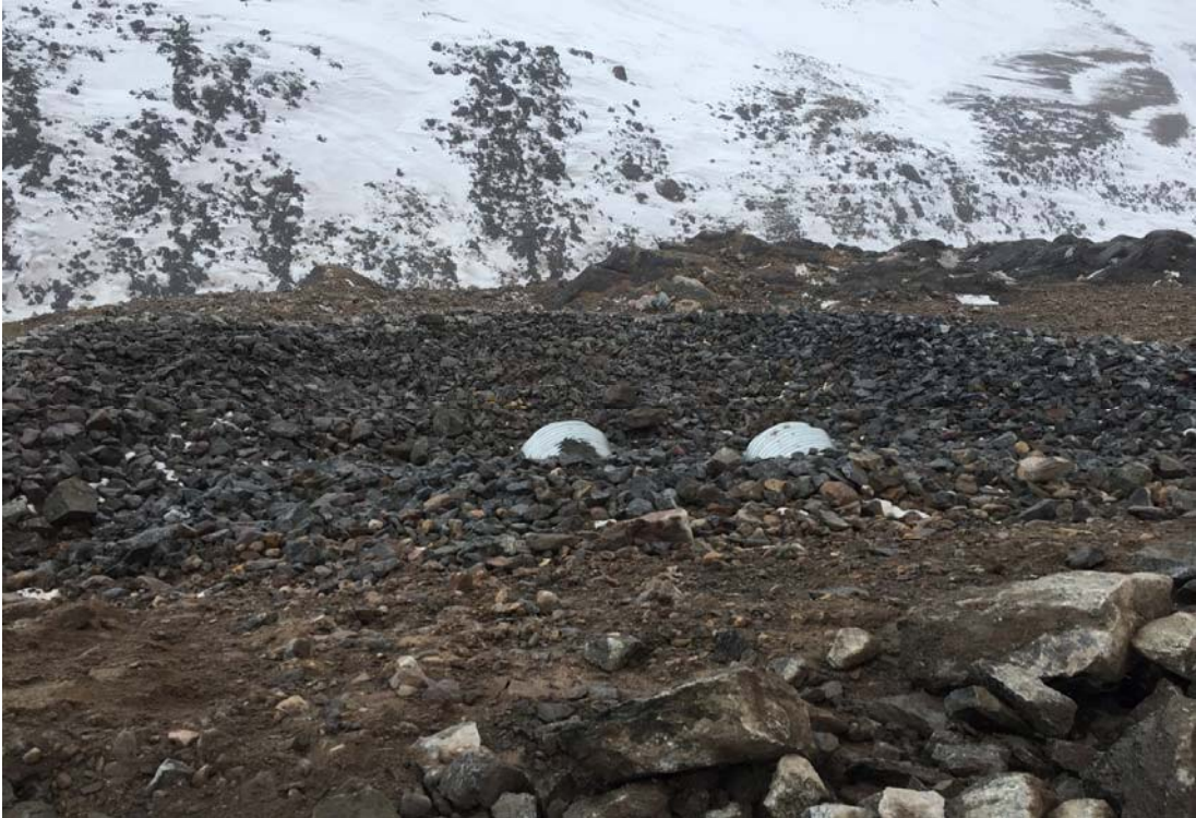
Culvert CV-1 Construction and Installation Photos – May 2016
