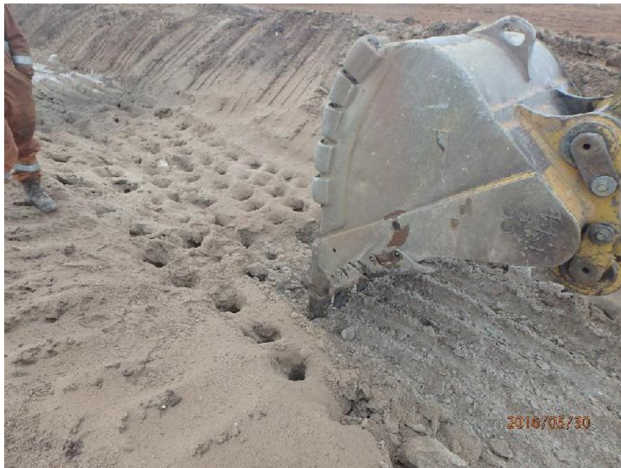
Figure 7: Excavator Bucket Ripping Pre Drilled Permafrost
