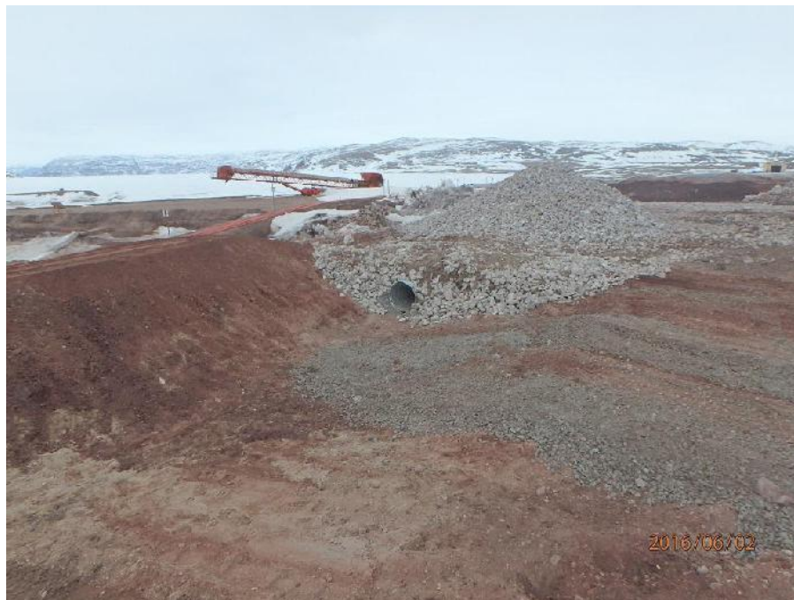
Figure 3: View looking North East with Swale, Berm and Back Filled Culvert
