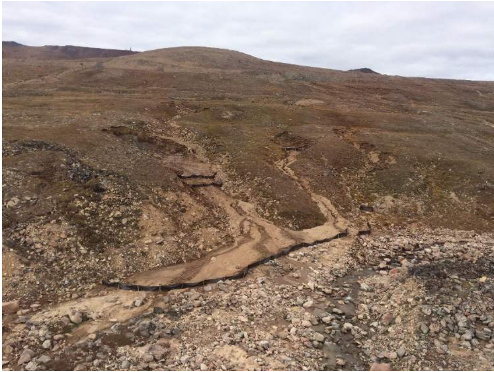
Photo 5 – Slope sloughing on MMER tributary upstream of Mary River with silt fence mitigation measures installed on August 26, 2016
