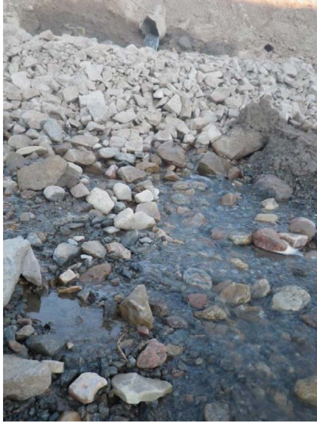
Photo 3 – BG-28 flowing clear at Km 86.5.
