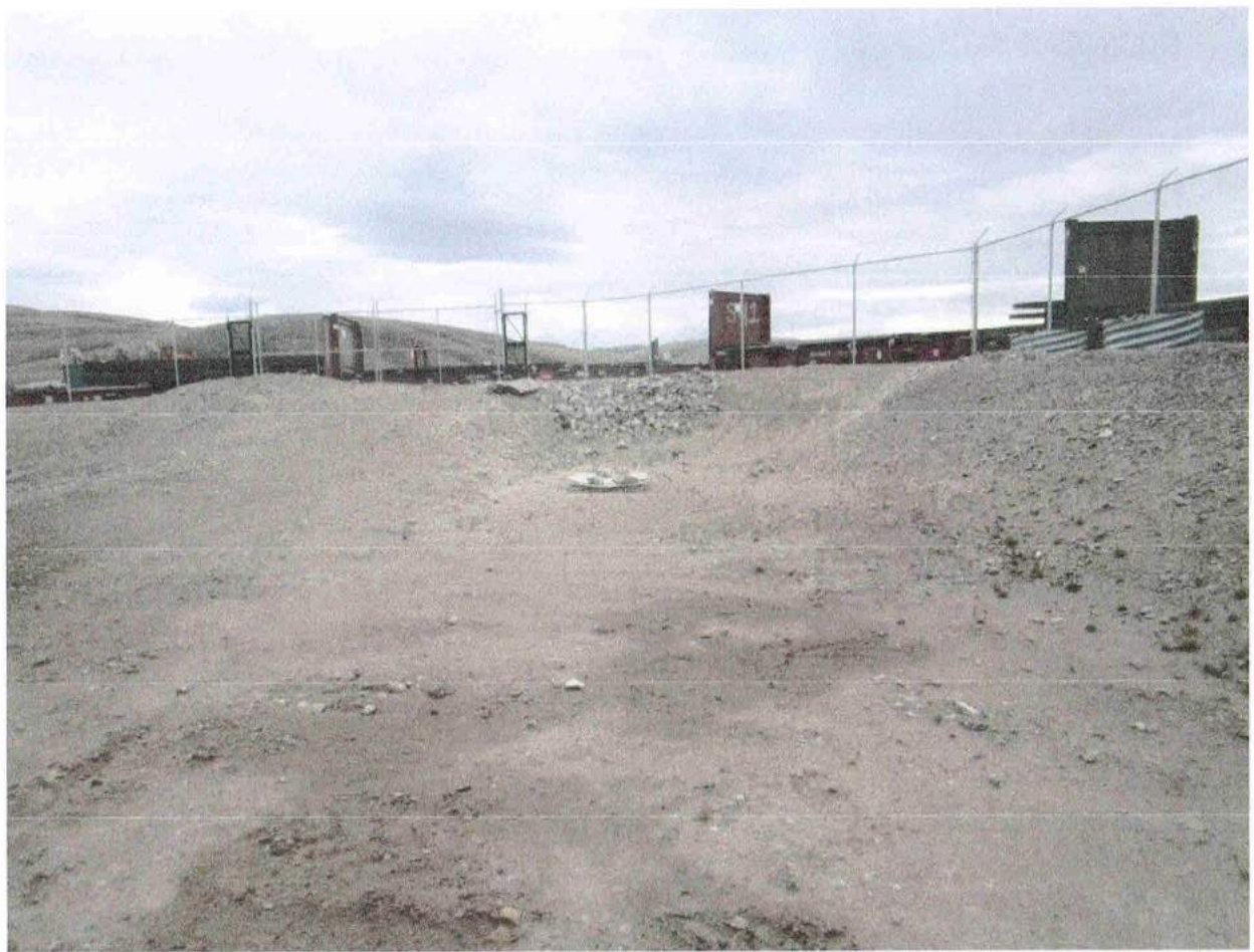
Fuel Tank Farm
