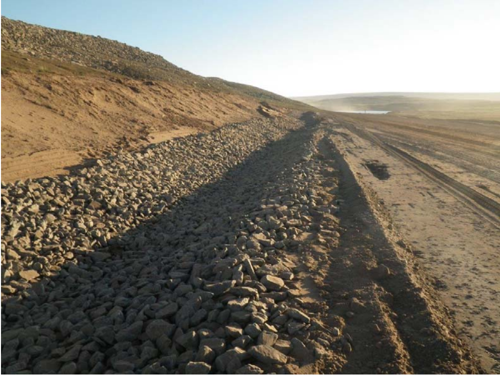
Photo 5: Rip rap in ditch at Km 85
