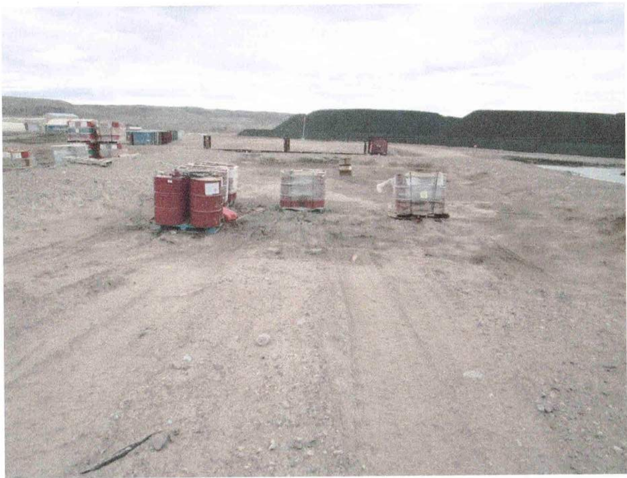
Hazardous Waste Storage MP-HWB-3
