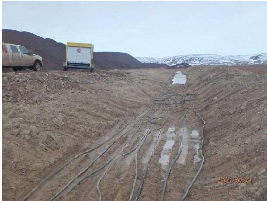
Figure 8: View showing Ground Thaw Unit being Prepared for Use
