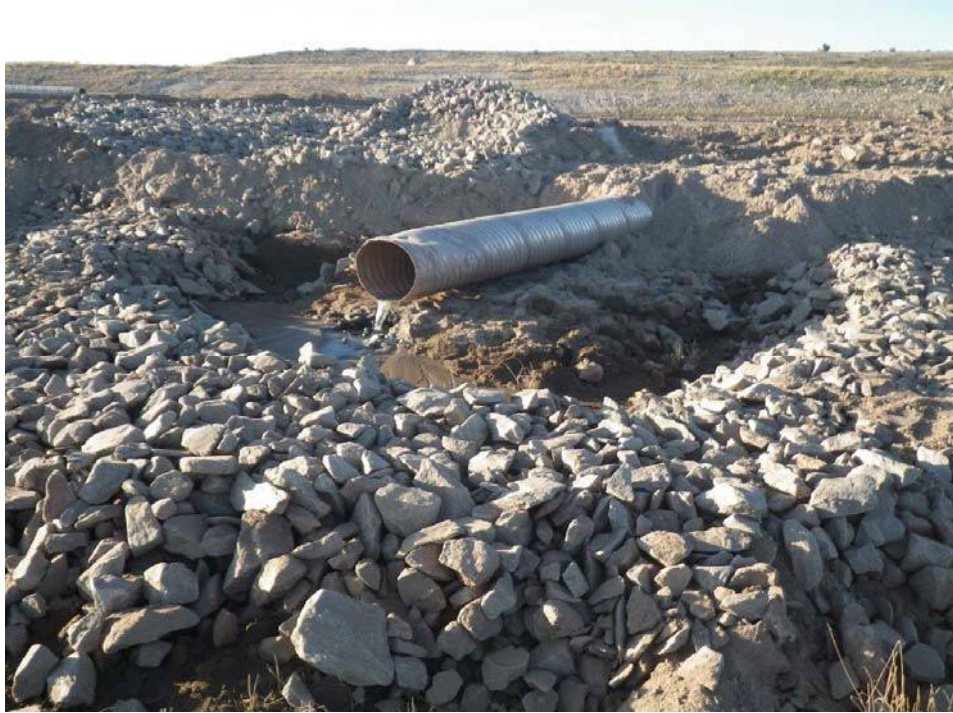
Photo 1 – BG-31. New culvert installation at Km 82 reduces siltation downstream
