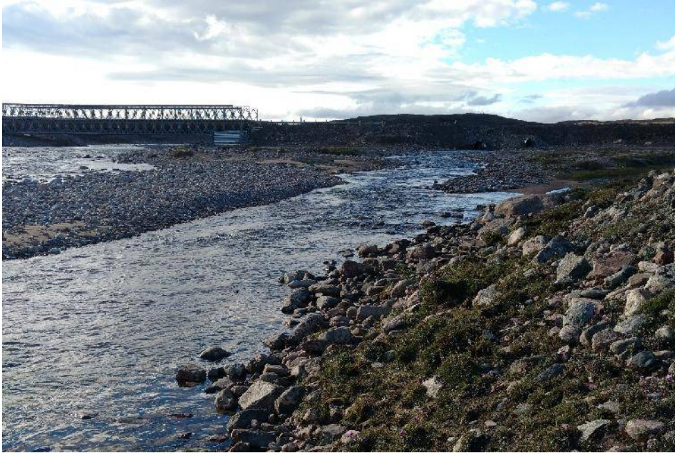
Photo 1 – Water flowing downstream of CV223 on July 31, 2016
