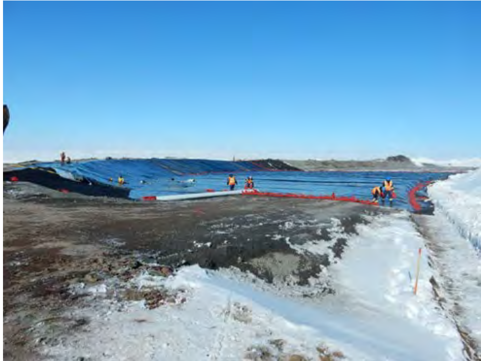
Figure 6: Liner Installation Nearing Completion
