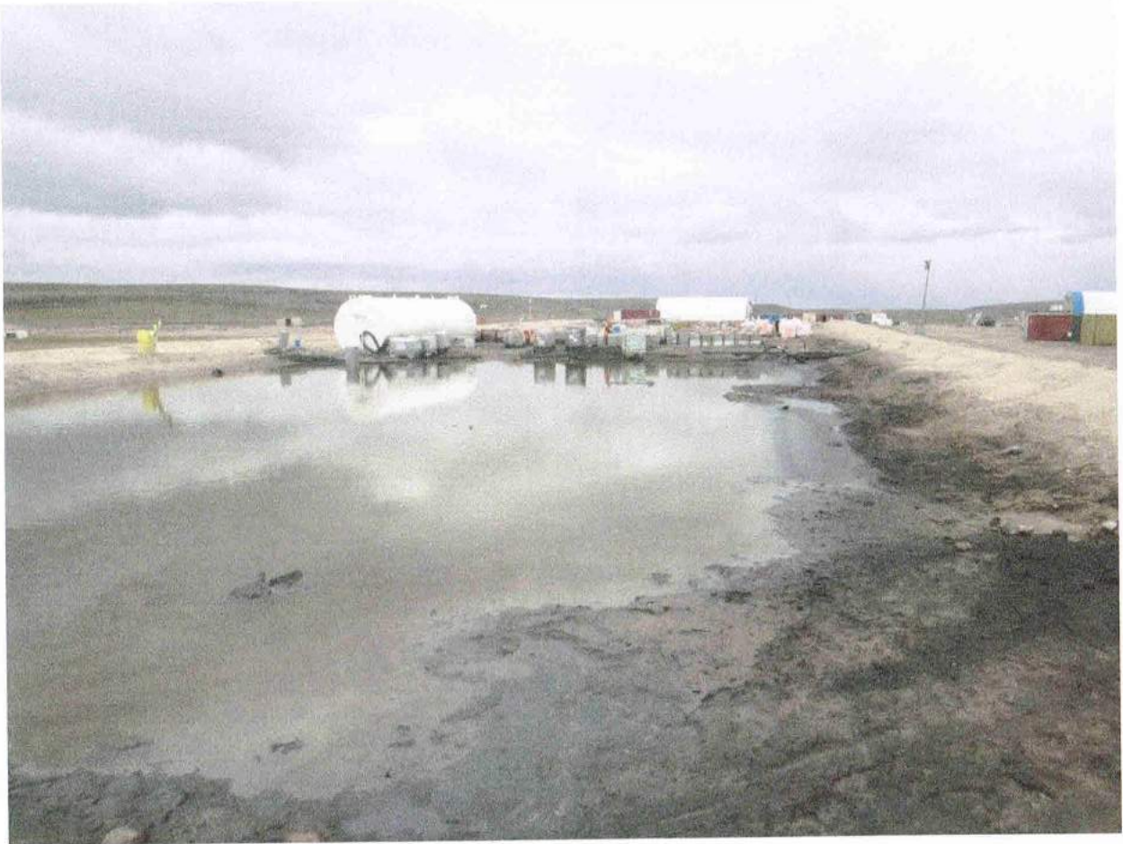
Bulk Fuel Storage Facility
