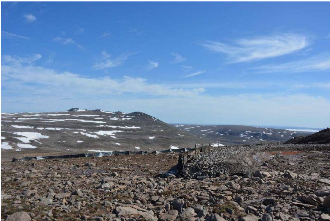
Photo 2 – Silt Fences and Checkdam #5 at Km 108.5. Picture taken on July 5, 2016.
