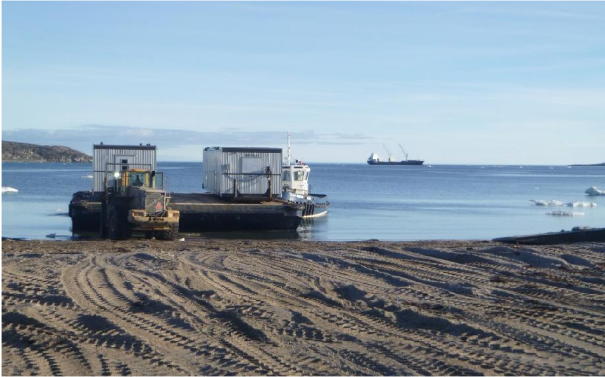
PHOTO 3 – Steensby Camp Structure Being Loaded for Transport to Milne Port, August 2016
