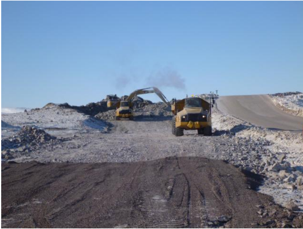
PHOTO 3 – Road Realignment at KM 53, May 2016
