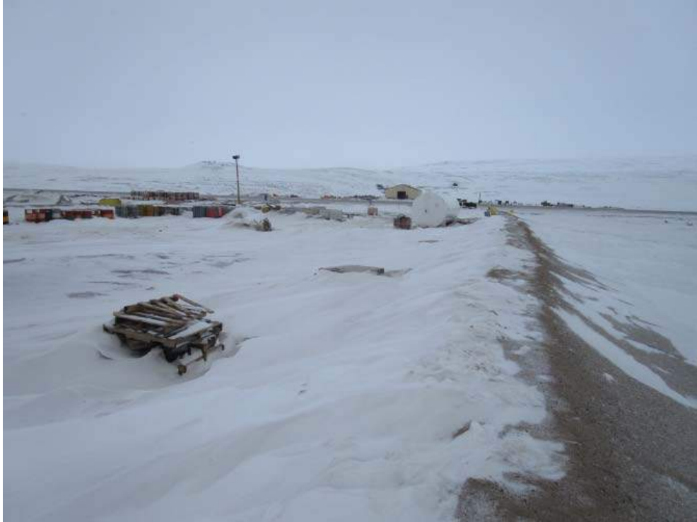
Bulk Fuel Storage Facility
