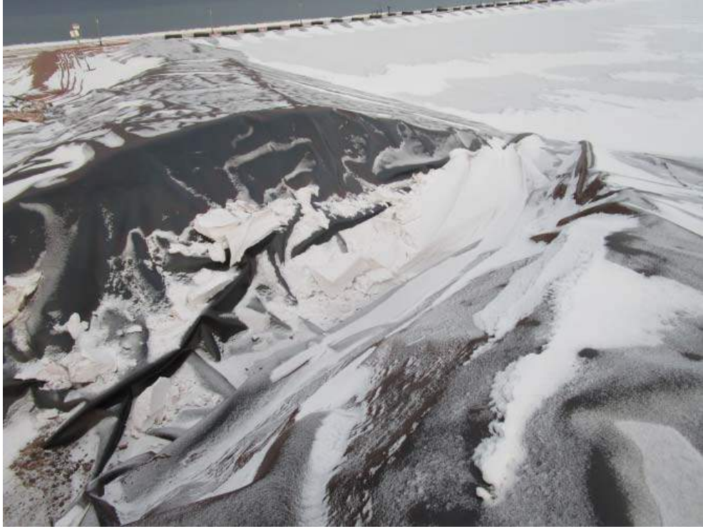
East Drainage Pond. Westerly Inlet
