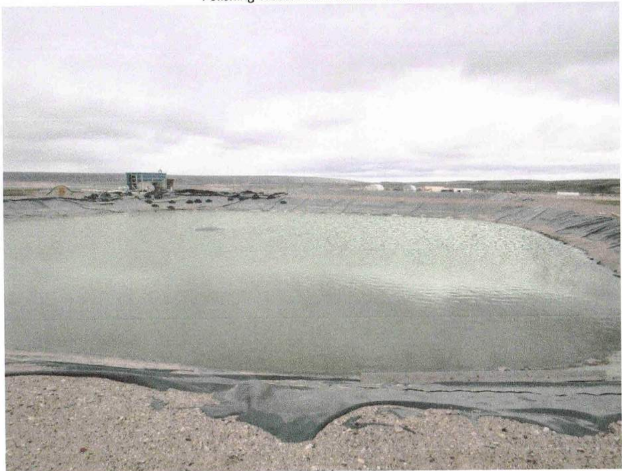
Polishing Waste Stabilization Pond #2.
