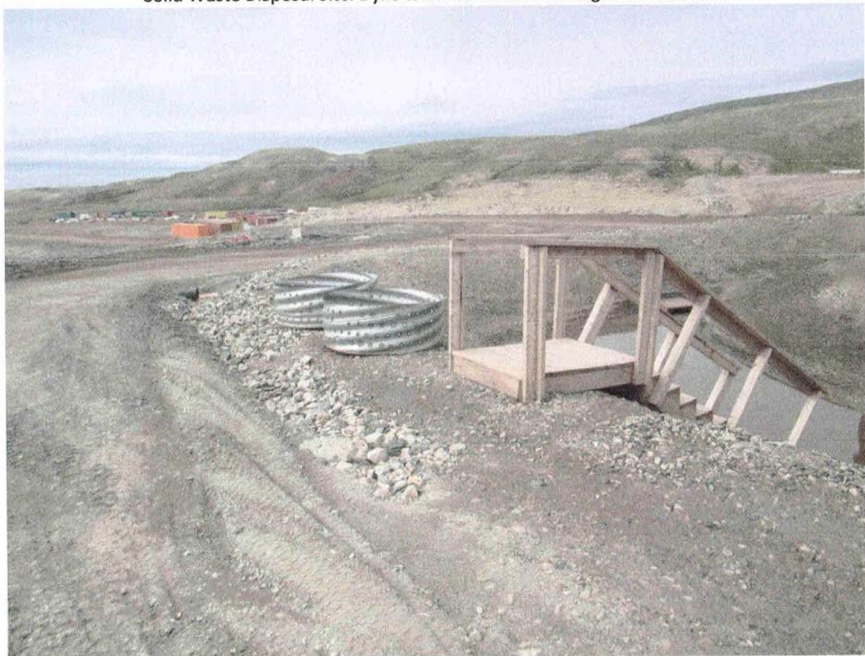
Minesite Steel Fuel Tank Containment. Sumps awaiting installation.
