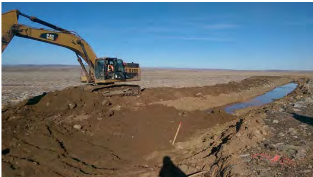
Figure 9: Ditch Excavation
