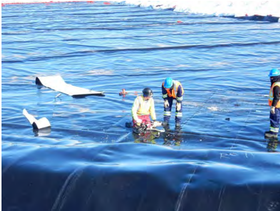
Figure 7: Seam Welding Liner
