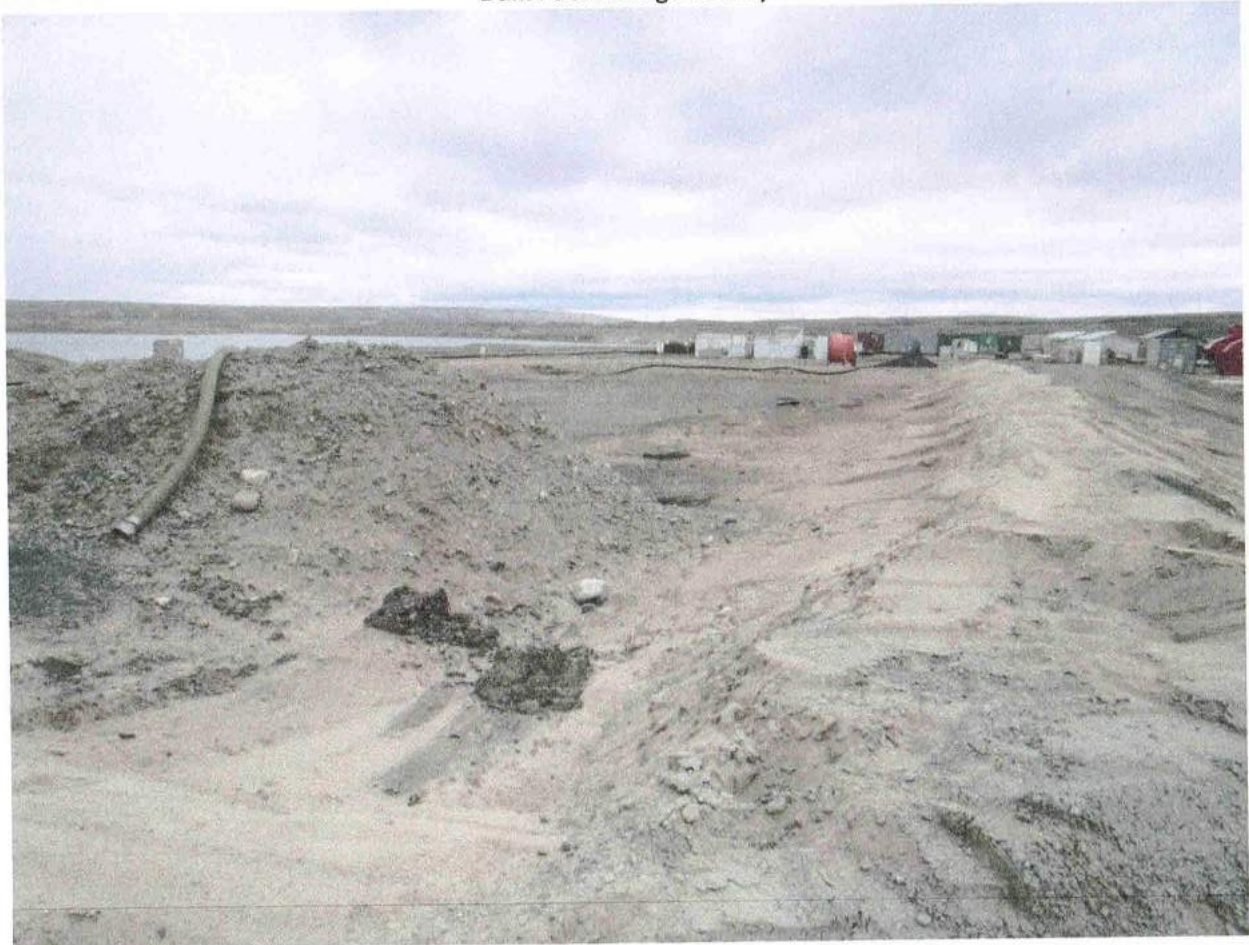
Generator Fuel Storage Facility. Containment now empty.
