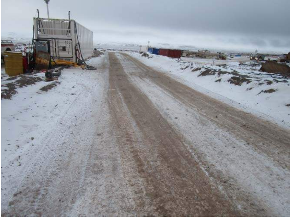
Fuelling Facility Containment
