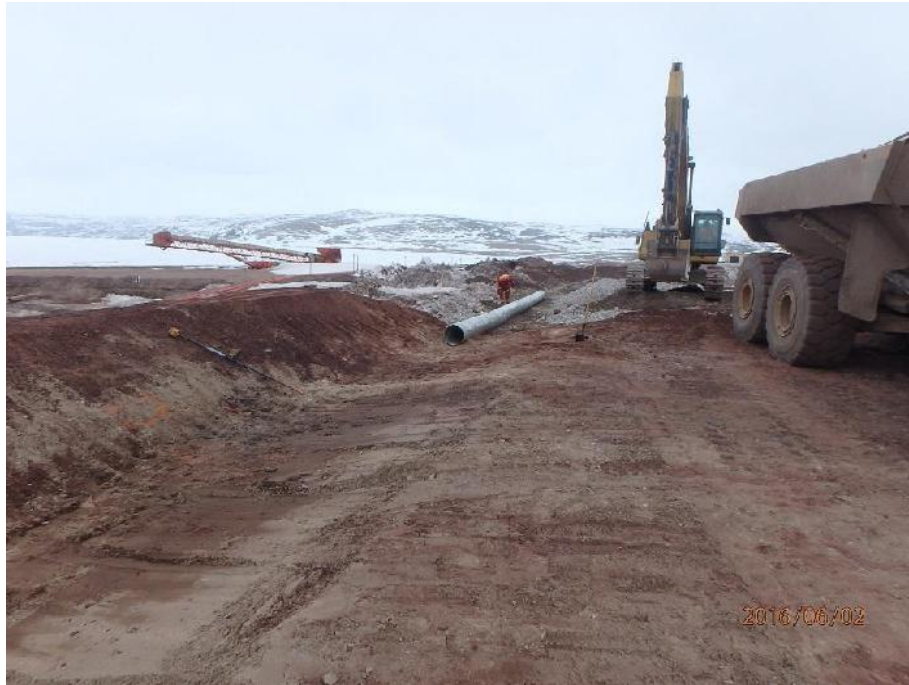
Figure 2: View looking North East showing Culvert being Placed
