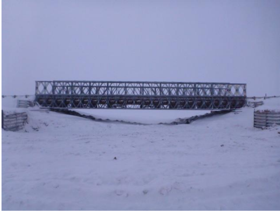
PHOTO 9 – Seacan Bridge Removed at Km 62, November 2016
