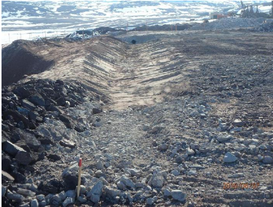
Figure 4: View looking East with Swale, Berm and Culvert
