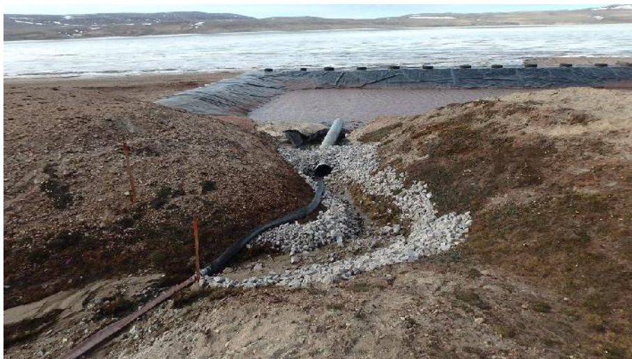
Figure 9: View looking North in to West Runoff Pond with Culvert Placed
