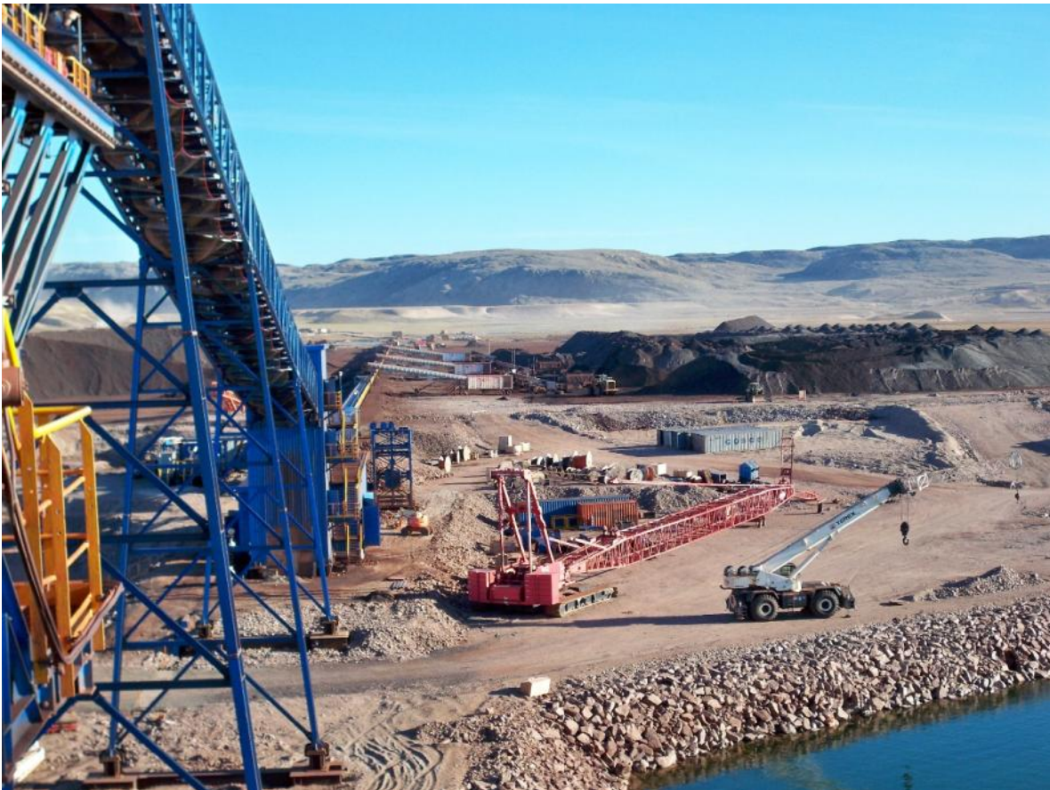
PHOTO 4 - Milne Port Ship loader Conveyor and Stockpile, 2016
