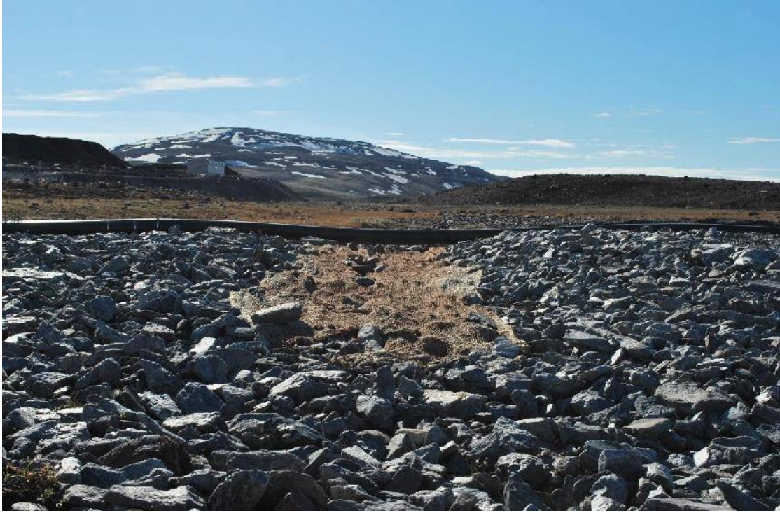
Photo 3 – Treated Jute installed at Check Dam #1 to capture sediments within runoff.
