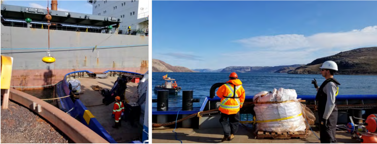
Figure 7: Equipment being lifted from the Milne Port Ore Dock to the Ocean Tundra (left) and the staging area on the back of the Ocean Tundra during deployment of Milne Port 01 mooring (right)
