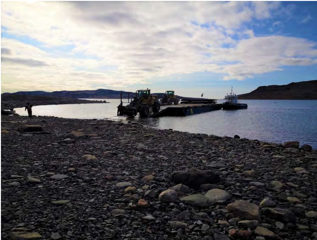
PHOTO 4 – Loader Coming Off a Lightering Barge at a The Sealift Landing Test Area
