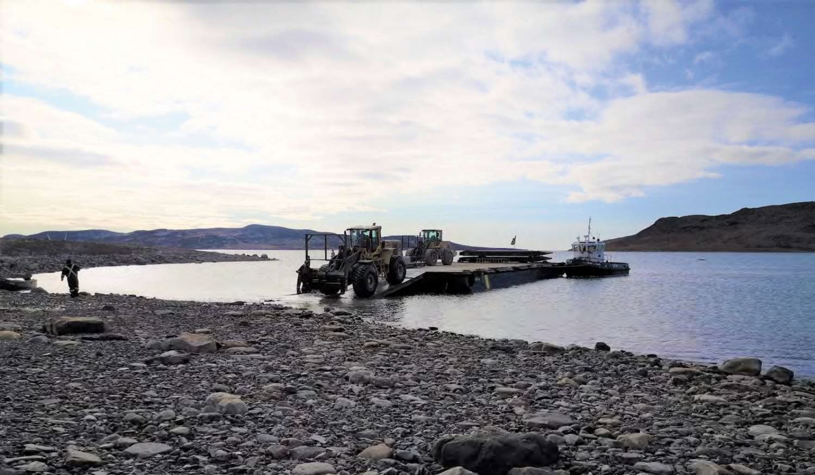
Testing the Potential Sealift Barge Landing Area
