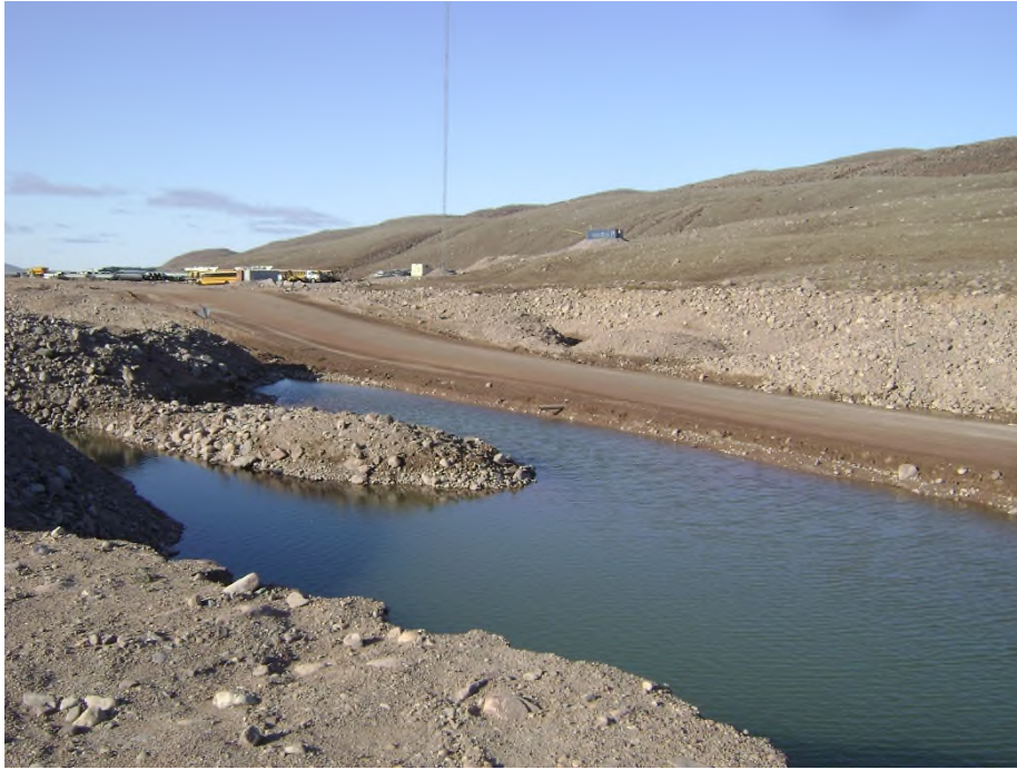
Photo 8 (2531): Pit at KM 7.2 with water on both sides of the new road alignment and extensive thaw of massive and wedge ice.
