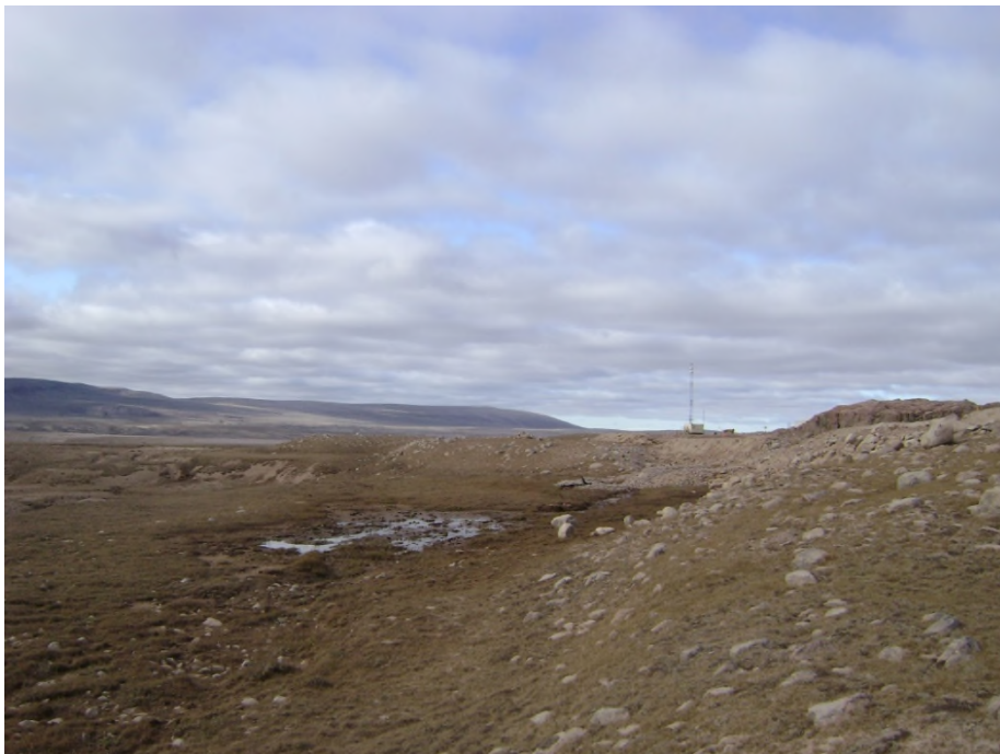
Photo 41 (2526): KM 4.0 erosion location. Photo shows wet area below the road on the top of the terrace.
