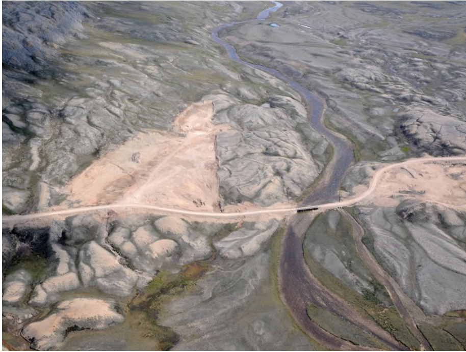
Photo 5 (DWH 2009 Photo 593): Pit at KM 61.7 (Figure 8) in 2009, compare to Photo 5A.
