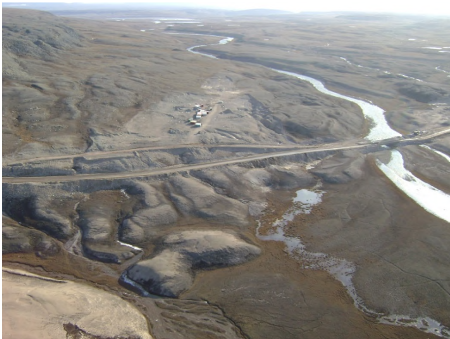
Photo 5A (2593): Pit at KM 61.7 (Figure 8), in 2014, note extensive settlement in southern portion (right side) of the developed pit indicative of the presence of massive ice in portions of this deposit. Note road realignment to improve grade.
