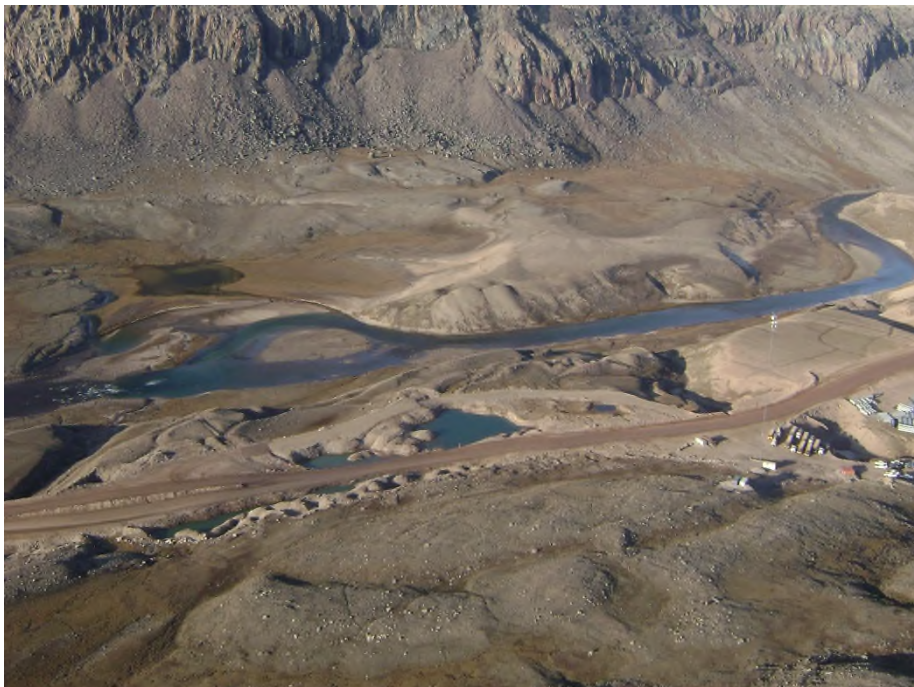
Photo 9 (2578): Pit at KM 7.2 – Note extensive thaw ponds on the west (right) side of the road. The road has been significantly realigned since 2014 and thaw has progressed dramatically since then. Road is likely founded on permafrost that contains massive ice thereby raising concern that thaw due to the ponded water could lead to failure.
